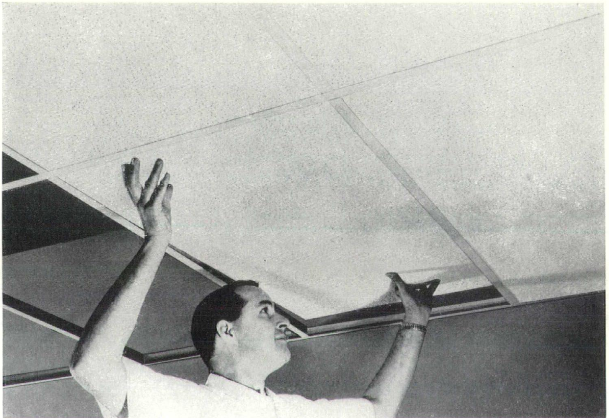
Large mineral fiber ceiling panels, capable of withstanding temperatures up to 2000°, quickly go into place in the Acoustical Fire Guard exposed grid suspension system. The panels rest on the supporting metal grids, and can be lifted out at any time for access to concealed utilities.
