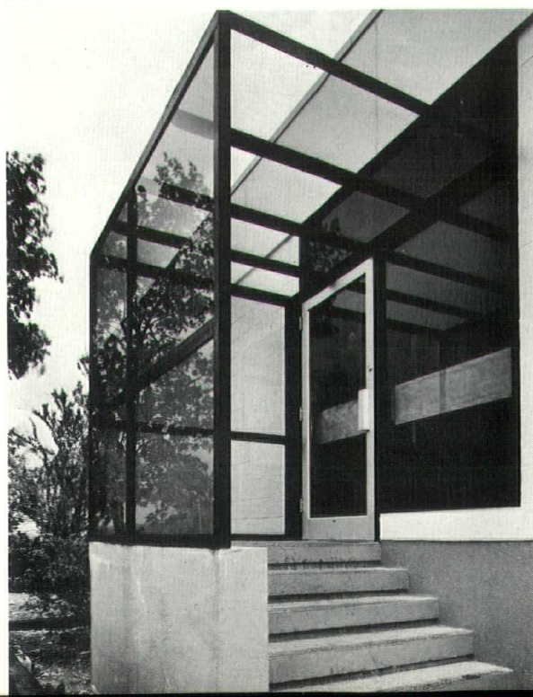
Structural system consists of long span steel joists on a structural steel frame.
