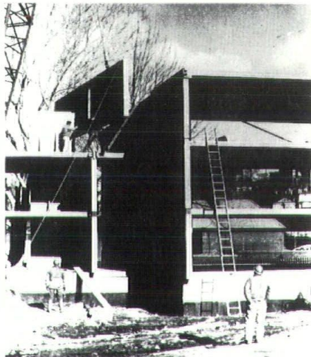
Precast concrete panels and hollow core slabs form system of construction for multiple unit housing project
