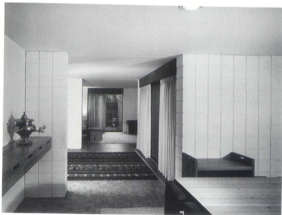
The masonry walls are load bearing with brick exterior and block interior.
