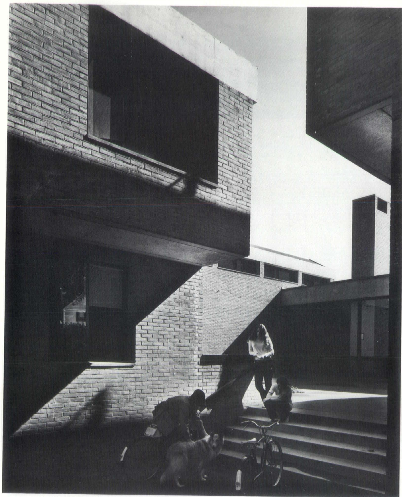
Load bearing masonry walls and concrete slabs were used throughout with exterior walls faced in brick.
