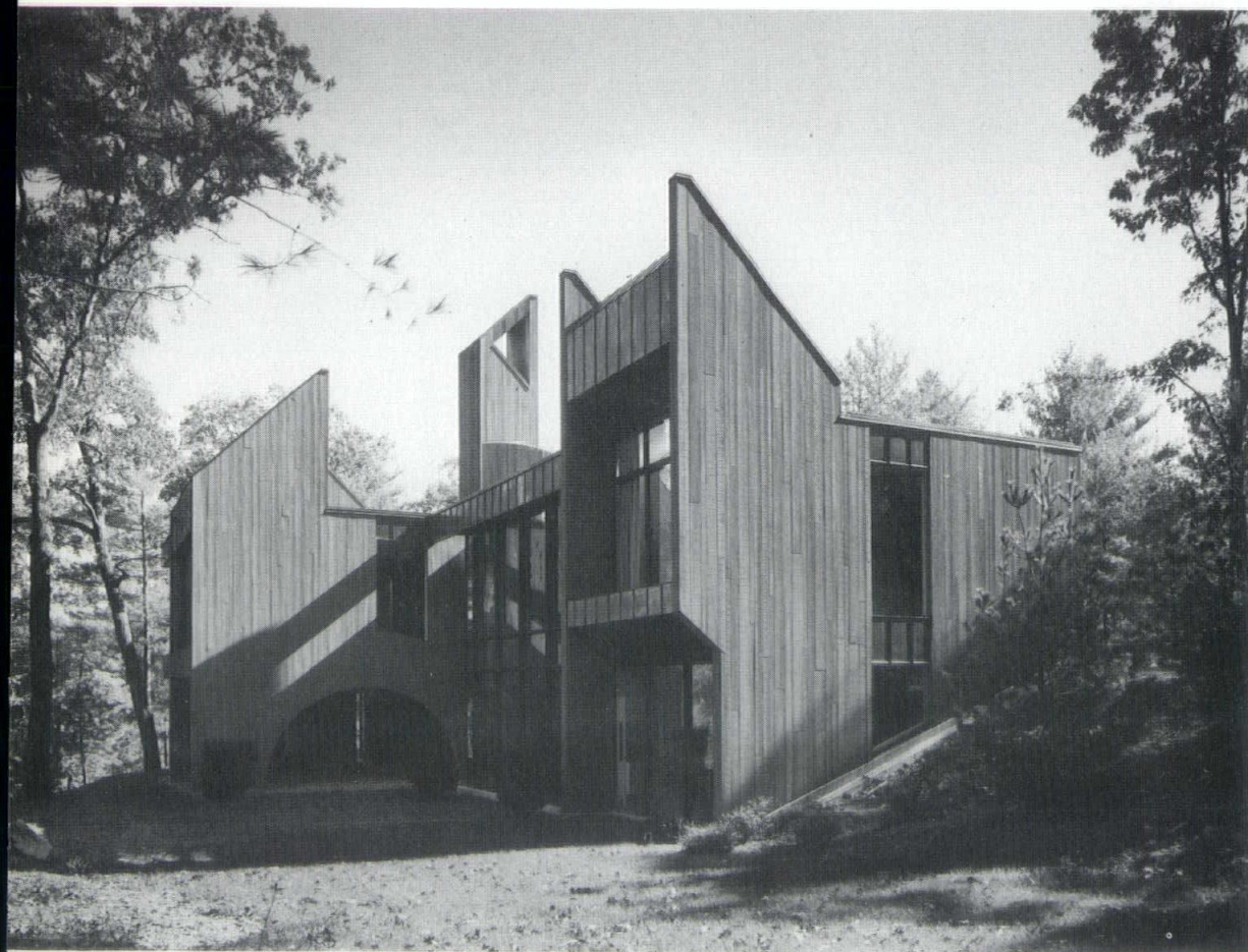
The rough-sawn, gray-stained vertical siding of cedar and extensive use of standing-seam copper are carefully related in color and texture to the lush site.
