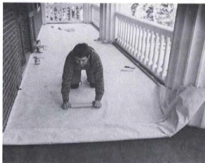
A rolling pin smooths out wrinkles.
