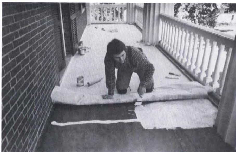
John brushes adhesive onto rough boards.
