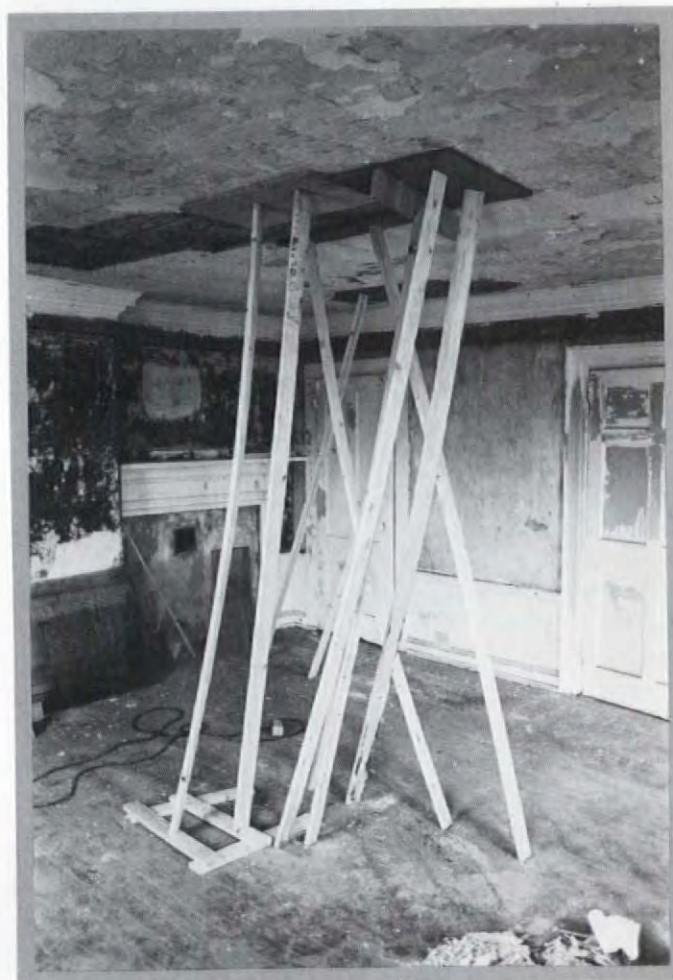
T-braces are wedged against the plaster to press it into place. Note the excess adhesive squeezing out.
