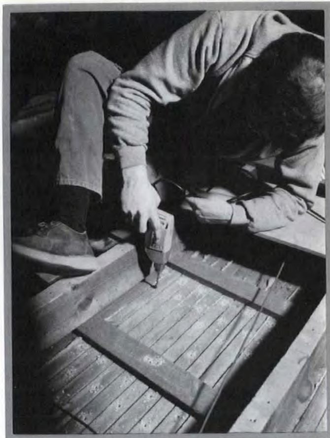
Use a drill stop on your bit to keep from drilling through the face of the plaster.
