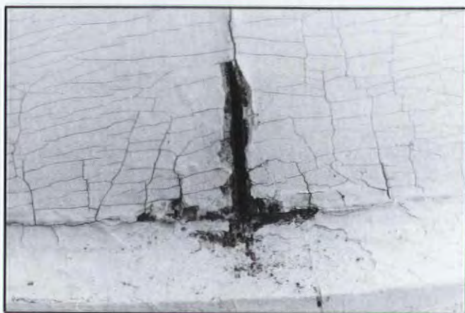
Vertical cracks indicate loose and open wood joints beneath the paint — movement is the culprit here.
