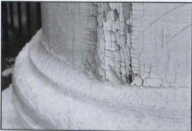
Alligatoring and cracking indicates the paint film is too thick. The remedy is to strip and repaint.
