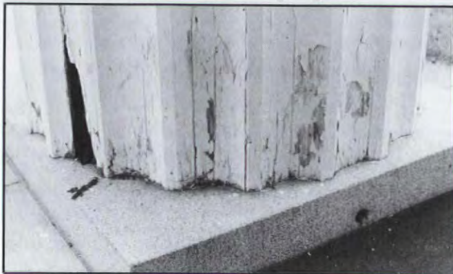
Paint failures tell their own story: Peeling down to bare wood indicates excessive moisture.
