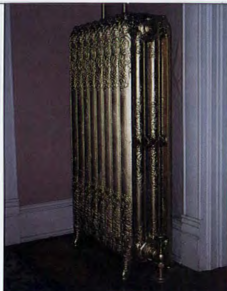
A finished rebronzing: dark pale gold on a 1910 ornamental rococo.
