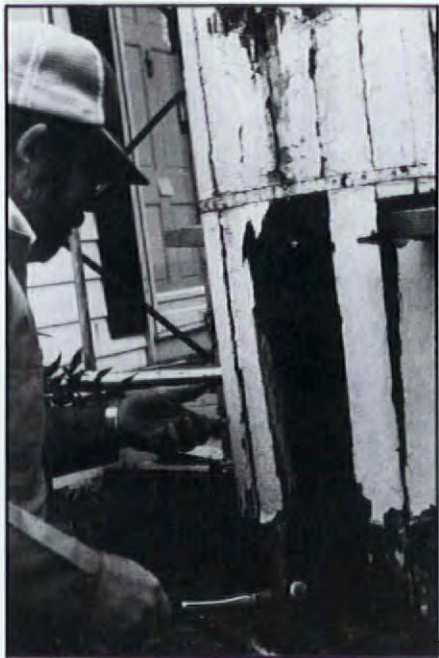
Removing the "worst case": Plunge-cutting the shaft makes room for a 2×4 handle. Then, by rigging with a block-and-tackle, the entire column is lowered to the ground.
