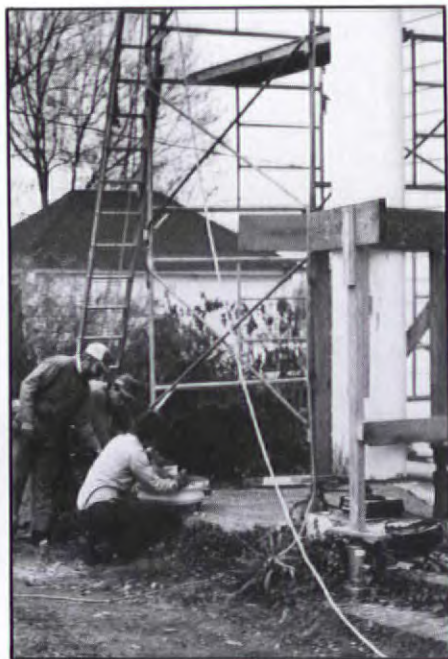
Three four-foot 2×10s bolted to each column (left), provided a triangular lifting jig for the hydraulic jacks. Electric heaters dried out the column interiors while the bases were patched and consolidated.
