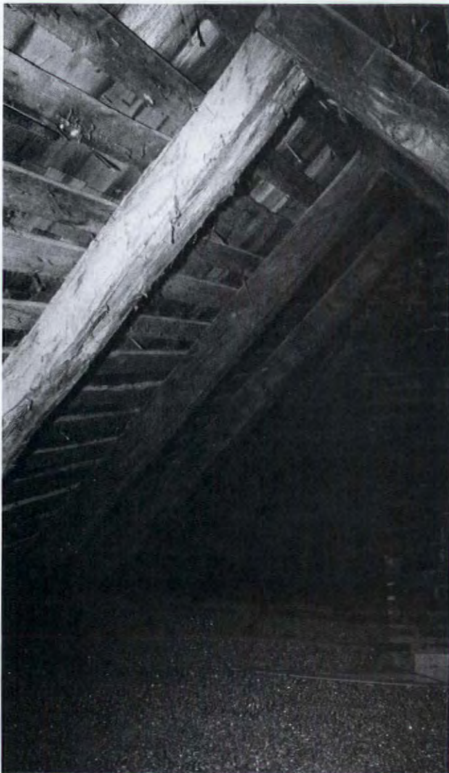
Old cedar shingles and nailing strips are visible in the attic. Over-roofing preserved the historic materials.
