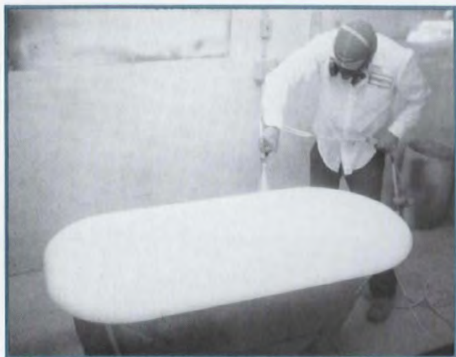
Polyurethane paint is sprayed on the carefully prepared tub in several applications.
