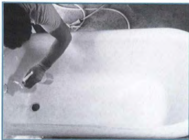
Phosphoric-acid cleanser in the spray bottle removes discoloration from superficial rusting.
