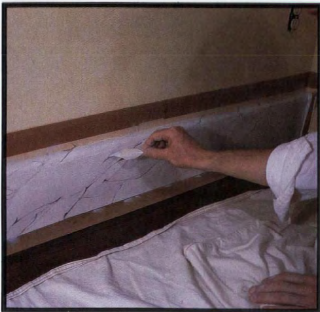
Black glaze is feathered on to create the white marble's fine veins.
