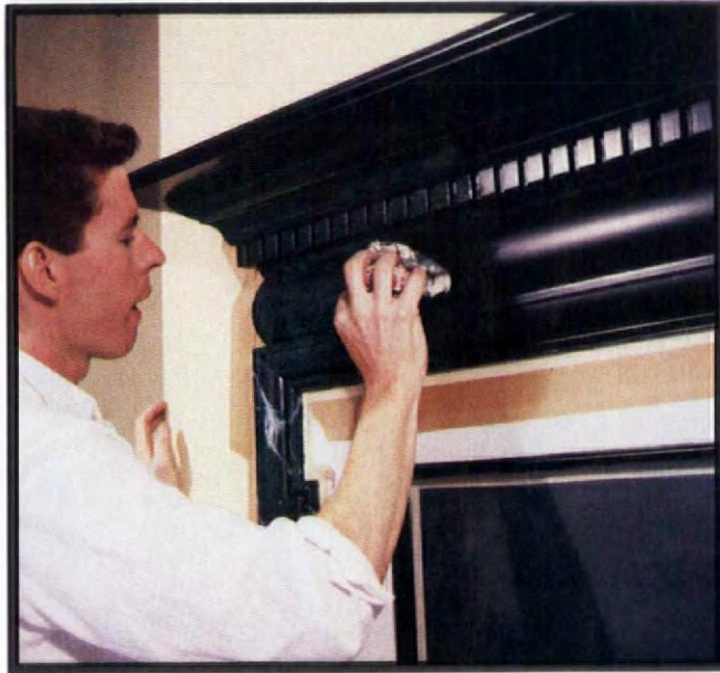
Ragging the undertone glaze with a bunched-up paper towel creates bare spots and shadows.
