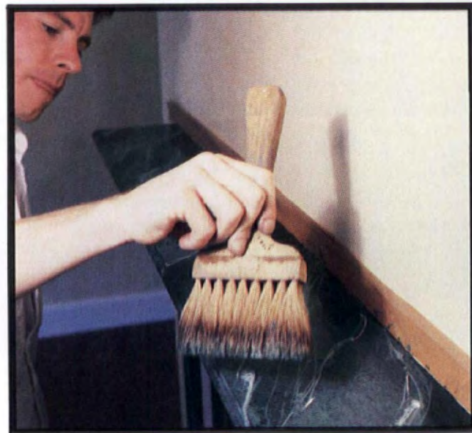
Jim "busbes" each vein before it dries with a badger blender brush to blur sharp edges and add depth.
