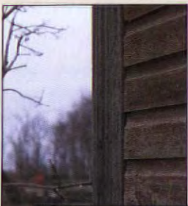
The ubiquitous "cove" pattern, also called "novelty" in its own right. Cove siding was popular by 1880, and may have been patented fifteen years earlier.
