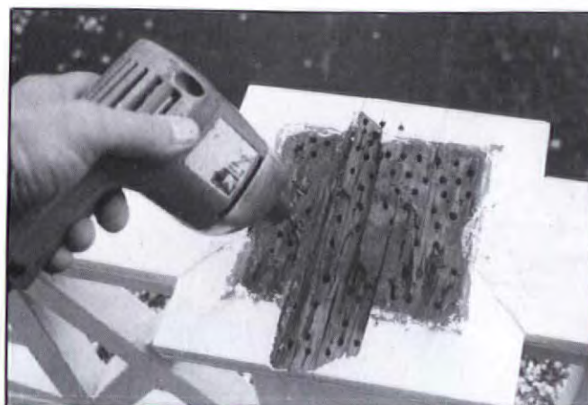
So that epoxy consolidant will penetrate, \frac{3}{16} " holes are drilled to just short of the underside.
