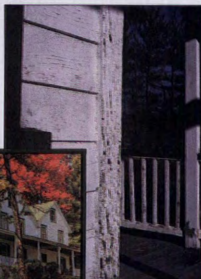
The Honold Homestead, Greeley, Penn. (c. 1880). Rectangular weatherboards, 4 1/2- to 5-inch exposure.
