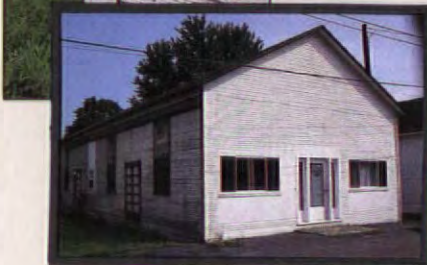
The ubiquitous "cove" pattern, also called "novelty" in its own right. Cove siding was popular by 1880, and may have been patented fifteen years earlier.
