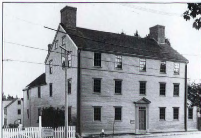
Typical practice on the New Hampshire seacoast: exposure graded from 2 1/4 inches at the bottom to 4 inches at the top (William Pitt Tavern, Portsmouth, 1766).
