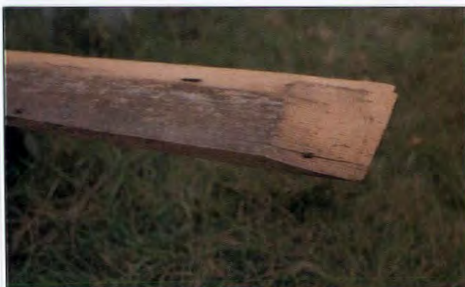
A hand-rived and -skived clapboard (Reuben Ball House, Corinth, Maine, c. 1808). Note the two-course nail holes.
