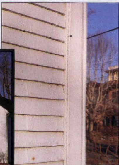
Silas Deane House, Wethersfield, Conn. (c. 1766). Skived clapboard, 3-inch exposure.
