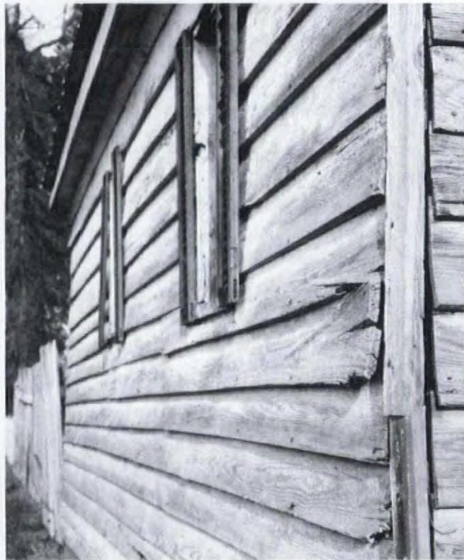
Horizontal lapped siding can often be rectangular rather than beveled.
