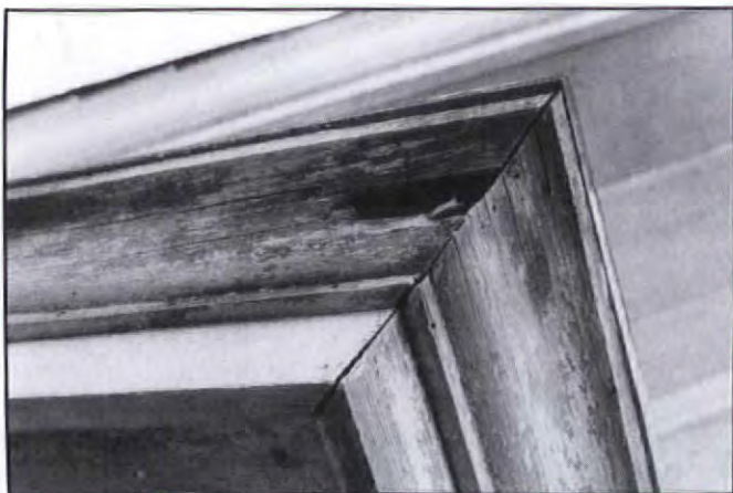
Treatment of this gable-end return cornice moulding will be easier if it's removed.
