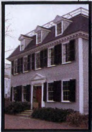
Henry Vassal House, Cambridge, Mass. (1746). Skived clapboard, 3 1/2-inch exposure.
