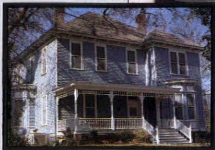
Henry Vassal House, Cambridge, Mass. (1746). Skived clapboard, 3 1/2-inch exposure.
