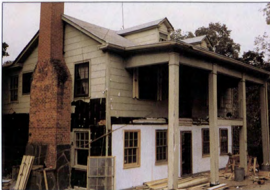
A major project was removing the asbestos shingles which had been placed on the house sometime during the late 1940s or early '50s.
