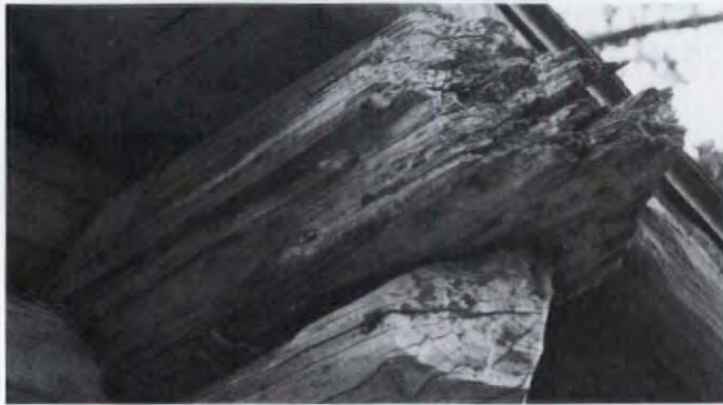
Typical severe deterioration of a log before restoration.
