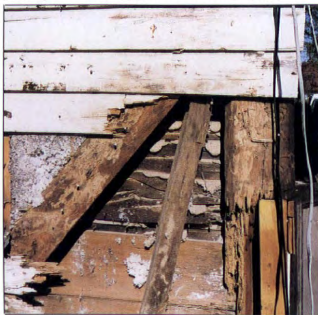
A close-up of the original shiplap and lathing chinked with Georgia clay and pig hair.
