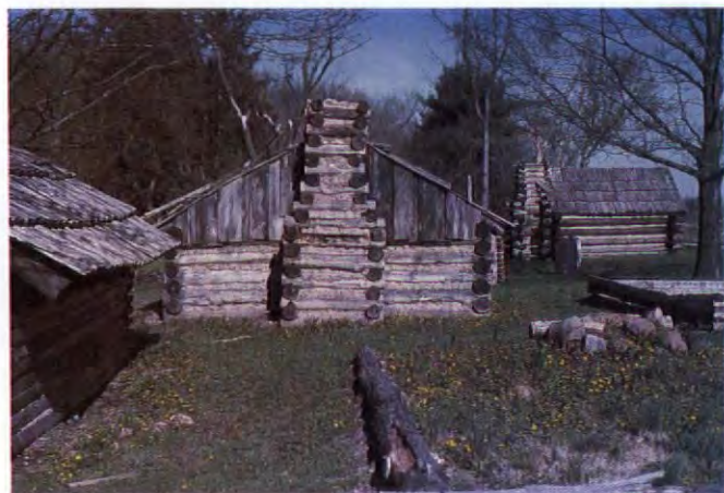
Reconstructed log soldier's but (Valley Forge, Penn.). Note log chimneys and in the round wall construction.
