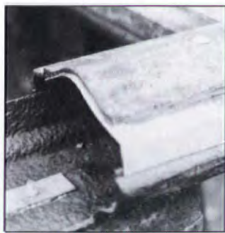
Ad-hoc reconstruction: A mending plate holds lower sections rigid; sheet steel is moulded for the top rail. Next, a salvaged top rail will be added and all the joints caulked.
