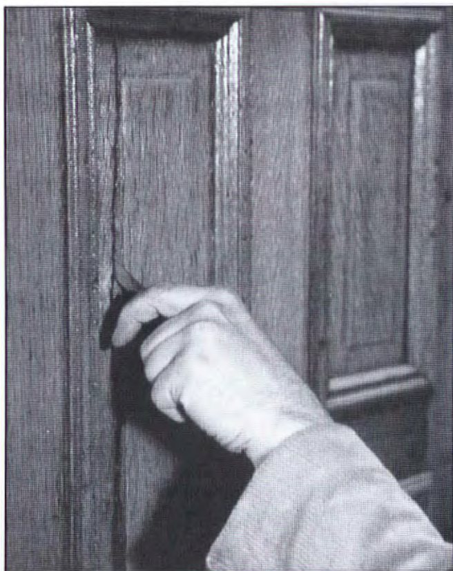
The opposite case: Although its split is long and old, the panel itself — which is still well-secured in the wainscot — is not in jeopardy.
