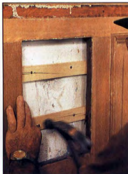
To reinstall a panel the same way, whole wainscot would have had to come off. Instead, a pair of short grounds were nailed to the wall.
