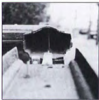
Ad-hoc reconstruction: A mending plate holds lower sections rigid; sheet steel is moulded for the top rail. Next, a salvaged top rail will be added and all the joints caulked.
