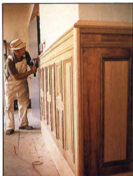
Missing panels: Cut on a table saw with an ordinary combination blade. After blade angle and depth were set, panel was run through on edge.
