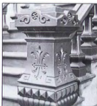
Paint layers build up; detail is uncovered by complete scraping, chemical removal, or sandblasting, which won't damage cast iron.
