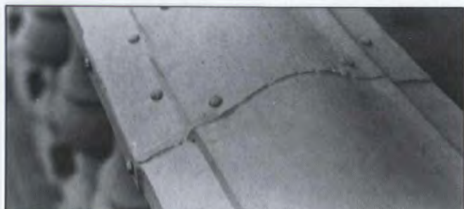
This sheet-metal patch, held by screws and caulk, are nearly 40 years old.
