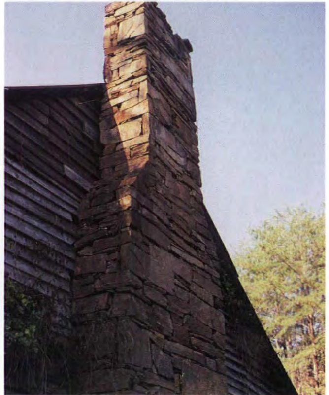
Note the tight, crisp, stonework of this single-shoulder, dry-laid chimney (Grayson House, Rutherford Co., N.C.).
