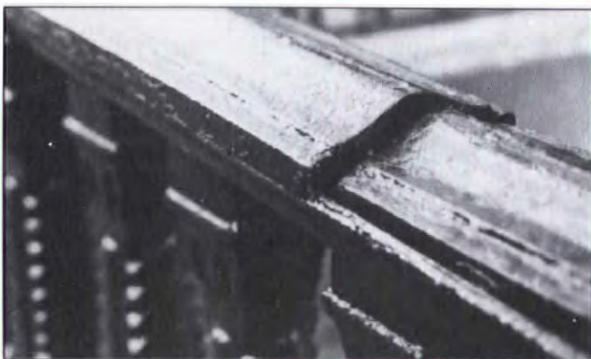
A segment of hollow rail has been displaced. The solution is realignment, a bolt through top and bottom of rail, and caulk between segments.
