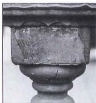
Paint layers build up; detail is uncovered by complete scraping, chemical removal, or sandblasting, which won't damage cast iron.
