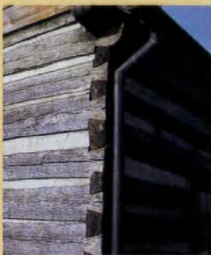
HALF-DOVETAIL NOTCH Smokehouse, early 1800s (Burke Co., N.C.)
