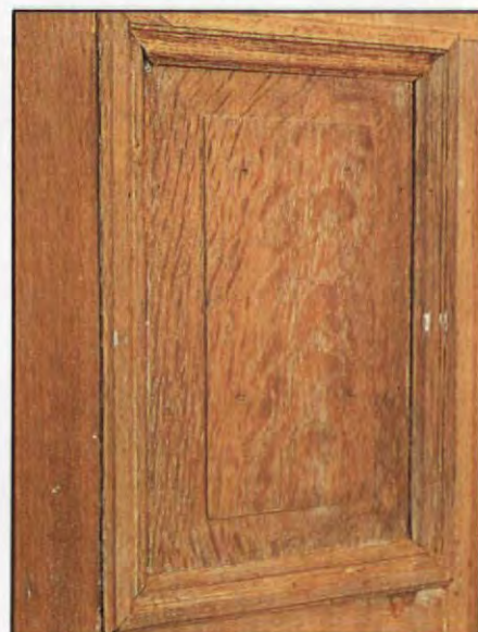
Completed panel was reinstalled with finishing nails, left and right, in pre-drilled bores. The panel floats and should survive another 100 years.
