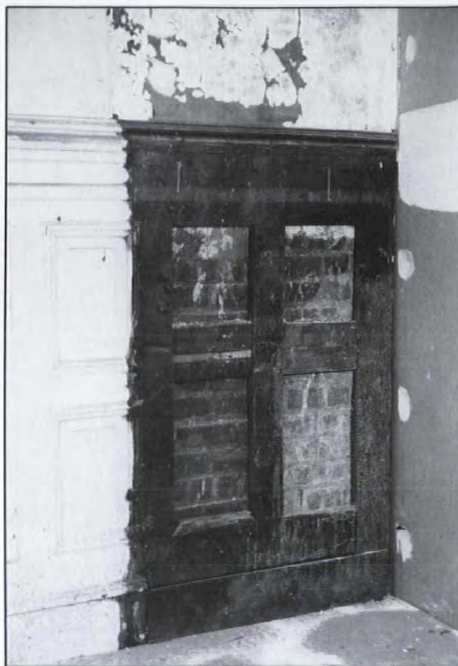
This panel framework is anchored directly to masonry. Panels, bolelection mouldings, and finish trim are applied later.
