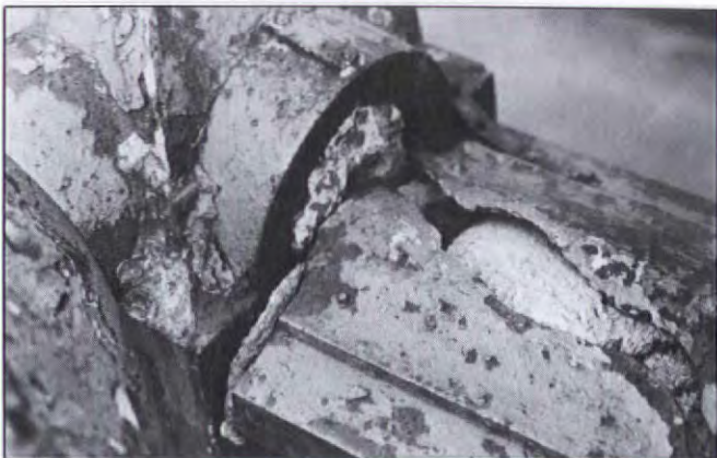
An example of exfoliated iron expanded by rust due to filling with concrete.
