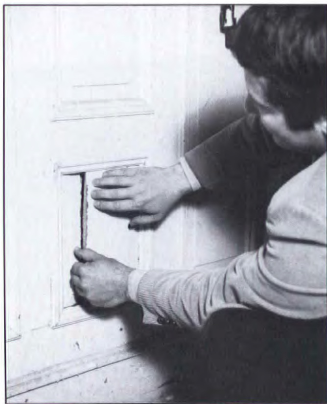
This panel had a hairline crack the owner may have been tempted to fill with paint. But a closer look showed it was completely unattached and ready to fall into the wall.
