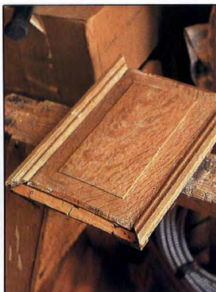
Applied panels were originally toenailed from the hidden side of the wainscot. Many were damaged by previous "restorers" prying them off.
