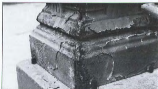
A professional repair job: The small tabs at the base of the newel are welded to the iron and set into holes in the masonry for stability. This is a shortcut job — the tabs should have been welded on the inside, where they'd be less conspicuous.
