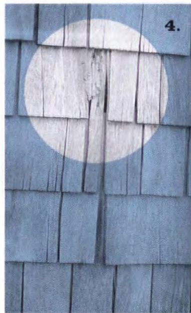
Sapwood decay has eroded enough of this shingle to expose the nail in the course below it.
