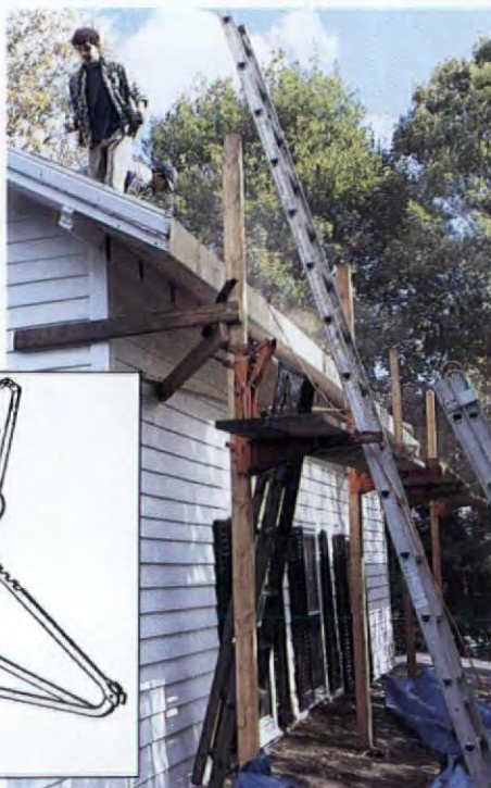
Ladder jacks (inset) will support scaffolding when used in pairs. Pump jacks (below) ride on 4 \times 4 columns braced to the building.
