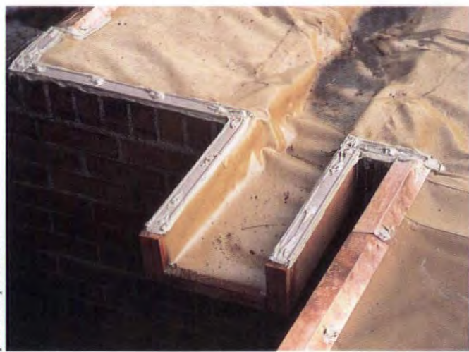
Water near the front doors was eliminated by taking the built-in drain over the brick wall and ending it at a scupper. Water spills into a gravel crock below, filled with 2" stone, Japanese Great Lakes in appearance.
