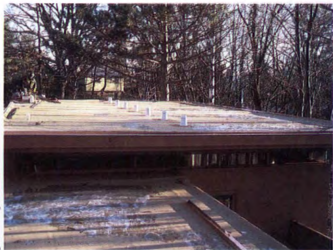
A roof, flat or otherwise, must breathe in order to last. The Duralast system includes venting boots to keep moisture from the bottom of the membrane. We used them to straddle each framing interval at the rafter, venting two joist spaces at the same time.
