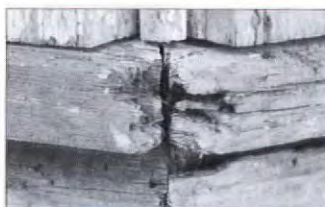
This rotted - and irreplaceable - woodwork...
