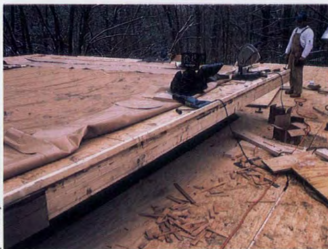
The membrane roof was on, above, but we went back when weather permitted to level and repair the fascia (see detail, page 44).
