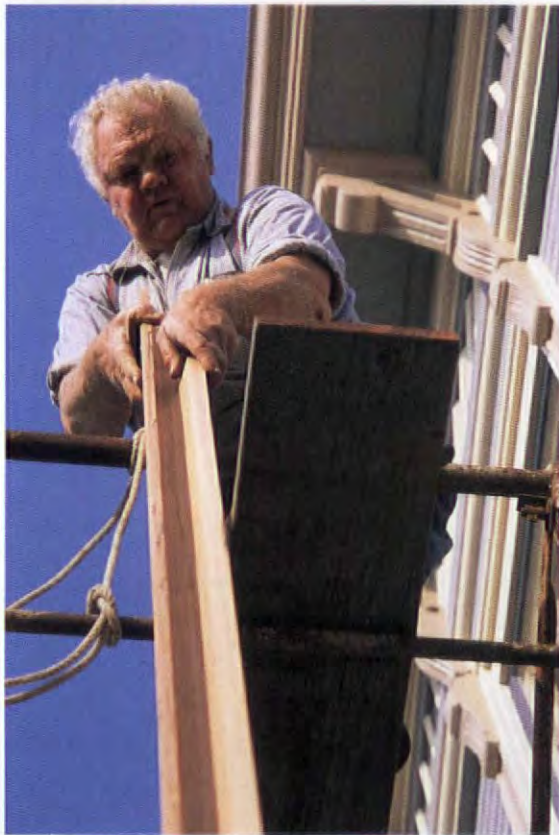
Top: Running a hose at the high point helps check the performance of this double-drain gutter installation. Bottom: new redwood gutter on its way to the eaves.
