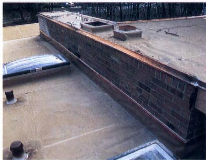
Above: a view of how the membrane is treated around the chimney flue as well as the copper cant and chimney flashing.
