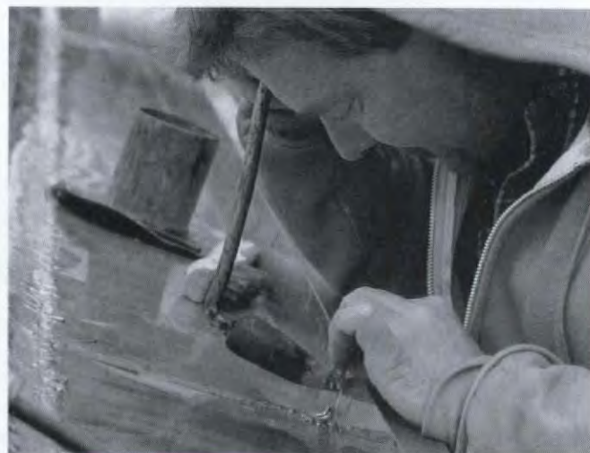
Soldering seams in a built-in copper gutter.
