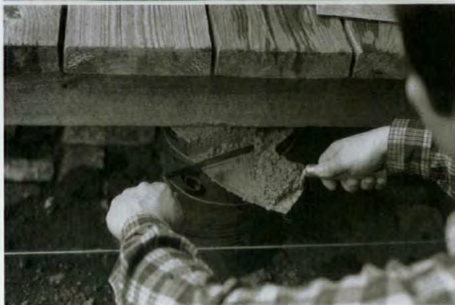
To fill a tube to capacity using a door, slide the door up the tube in stages as you add concrete mix (top), then top off the tube when the door is at its maximum height (above).
