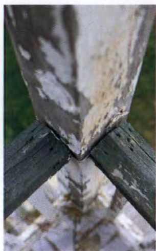
Shifting of the porch opened these toenailed rail joints, allowing water to enter and weaken the ends.
