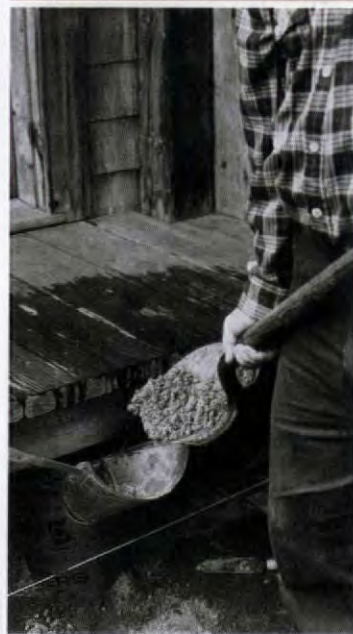
When working solo on a tube with blocked access, hold the fill funnel in place with improvised straps.
