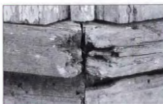
This rotted - and irreplaceable - woodwork...
