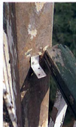
Knee plates mount to the porch support first. Then the rail (mortised at the end to accept the plate) is angled on and attached from below.
