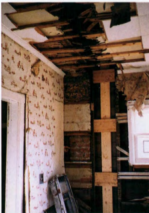
Above: our "mobile home" en route. Left: Here's how our kitchen looked — note the severed furring — after it was joined to the rest of the house.
