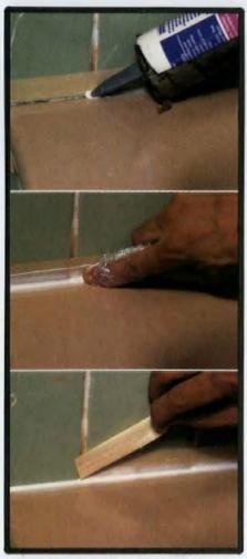
Top: Mask the joint at the appropriate bead size and gun in caulk. Middle: "Tool" the bead so caulk is thinnest where it meets the tape. Bottom: Remove the tape immediately, before caulk skins over (bottom).
