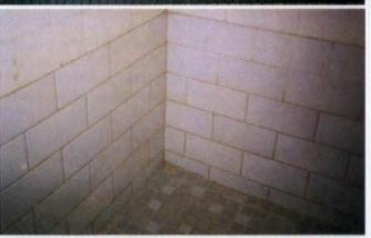
Top: Our 1"-square replacement tiles closely resembled the shower floor's original ¾" tiles. Middle: When retiling the shower curb, we couldn't locate step tiles of the proper thickness, so we used cove and wall tiles, trimmed to fit. Bottom: Our new white wall tiles made us more appreciative of the original ivory ones.
