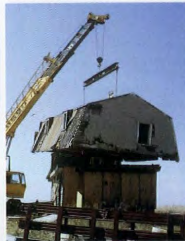
The Cook House had to be sectioned in order to make its 125-mile journey practical. Left: removing the roof by crane. Right: cutting away the added wing.
