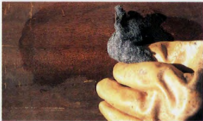
The new alternative strippers require time to work and generally have the easiest job on simple, clear finishes.
