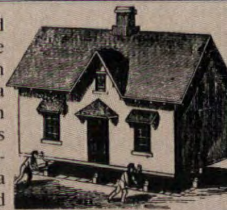
Raising with screw jacks, c. 18
