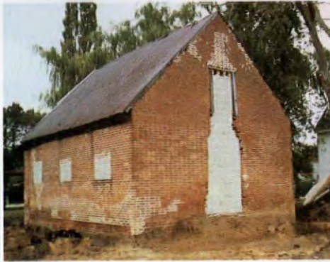
Preparing the stable by blocking in wall voids and excavating the foundation.
