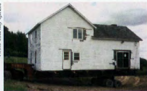
"Going three points": two dollies (at rear) and the tractor's fifth wheel.
