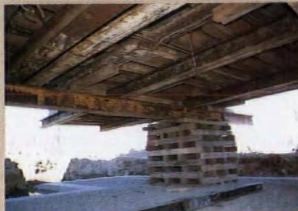
Once off the foundation, the building sits on a network of steel beams.
