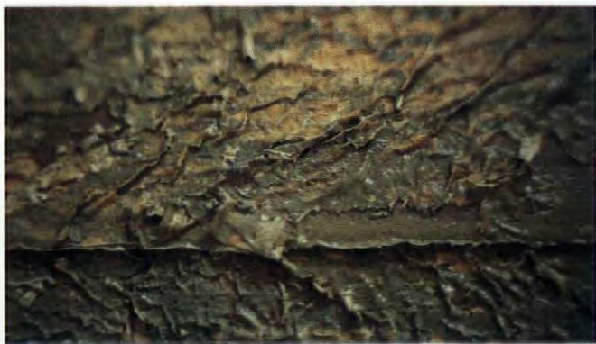
Swelling and bubbling of the paint film characterize solvent-based strippers containing methylene chloride. Covering the stripper with Saran Wrap or wax paper while it works will contain solvents and coax more effect from stripper.
