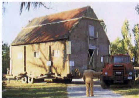
The solid-brick stable moving off the old foundation and onto the road.
