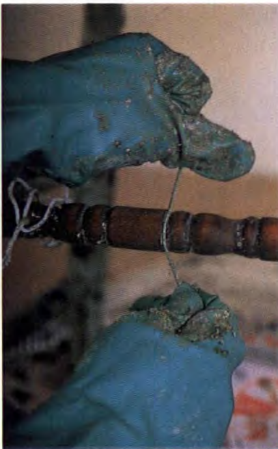
Strong twine helps remove softened paint sludge from baluster or furniture turnings. Chemical-resistant gloves should be worn.
