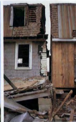
The Cook House had to be sectioned in order to make its 125-mile journey practical. Left: removing the roof by crane. Right: cutting away the added wing.
