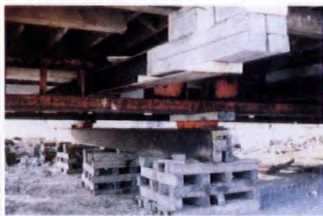
Skate dollies riding on steel may be used for short moves.
