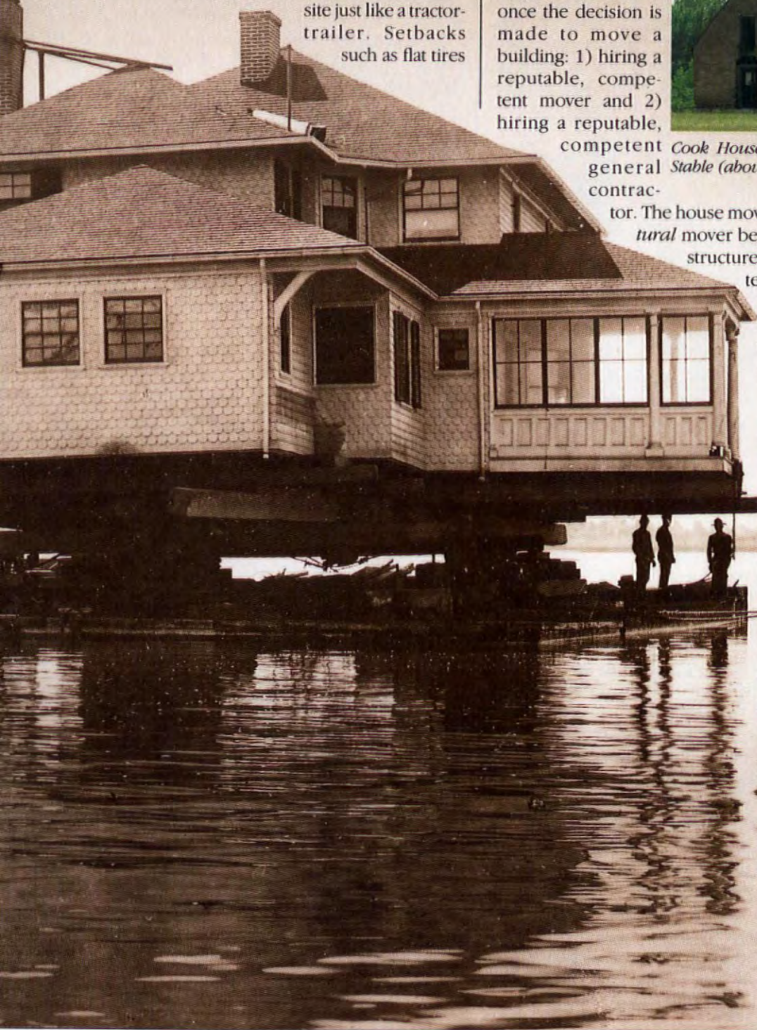
House moving by water from San Diego to Coronado, Calif., in the 1910s.
