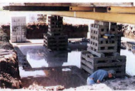
Footings may be pre-poured, but most foundations are built up to the house.
