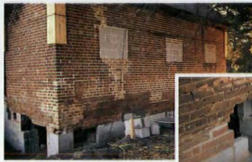
A new foundation and holes left by steel.
