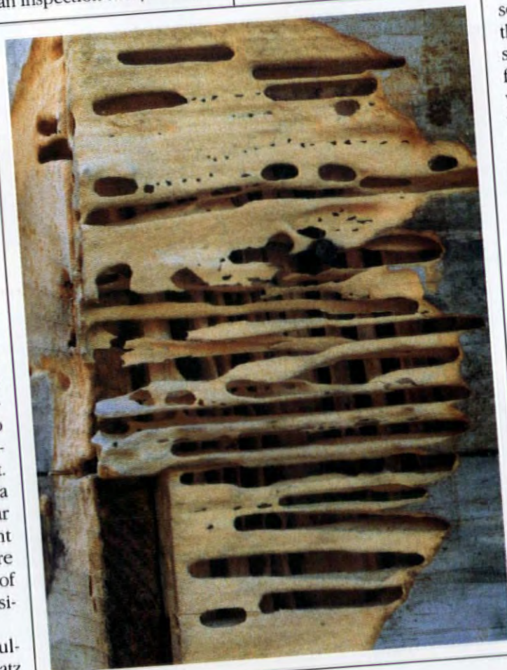
Clean, smooth-surfaced galleries chewed out of softwood sheathing — the nesting place of carpenter ants.
