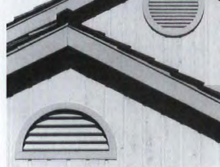
All Sammamish's gable vents have a stout mesh back for insect control.
