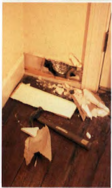
Top: newly peeling paint, a telltale sign of wet plaster. Above: Water-soaked wall insulation can be located and removed by carefully prying off baseboards.
