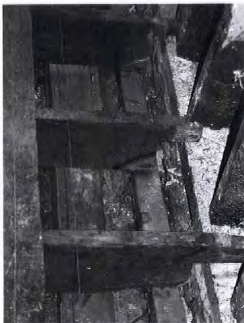
Weakened masonry and framing typical of the ailing substructure we found in areas around the building.
