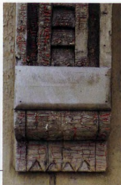
Far left: Peeling down to bare wood may be caused by water-vapor migration. Left: Poor preparation can lead to peeling between coats.
