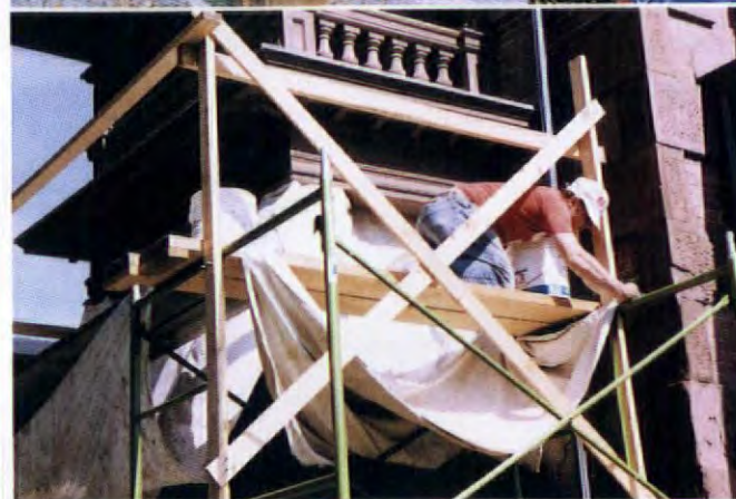
Top: Anne-Marie Lord prepares a wood balustrade by stripping heavy sanded-paint buildup with steel scrapers (which must be resharpened frequently) and a chemical remover. Above: Safe, stable scaffolding allows the team to concentrate on the sanded paint. Tarps control drying and overspray.
