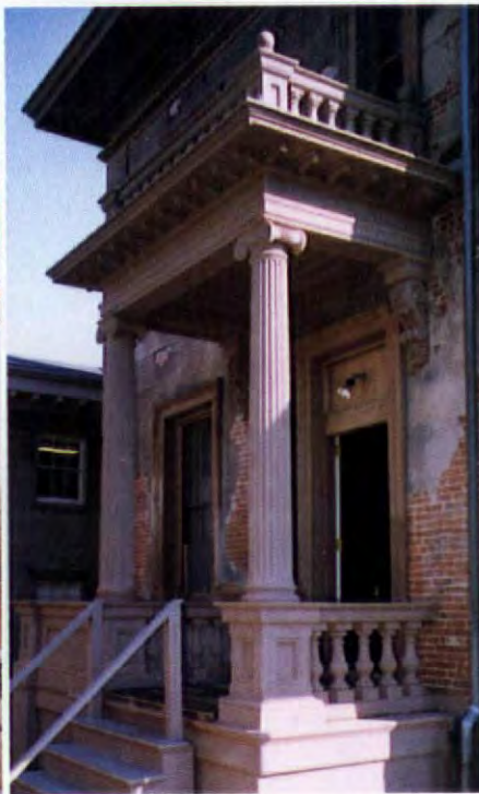
The Victoria Mansion (left) was built of brick faced with brownstone in the Italianate villa style. Appendages such as the rear porch (right) were constructed of wood and then finished with sanded paint to match the stone veneer.
