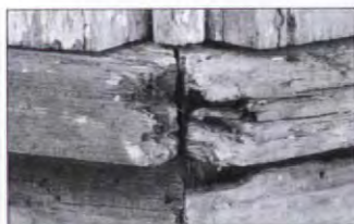
This rotted — and irreplaceable — woodwork...
