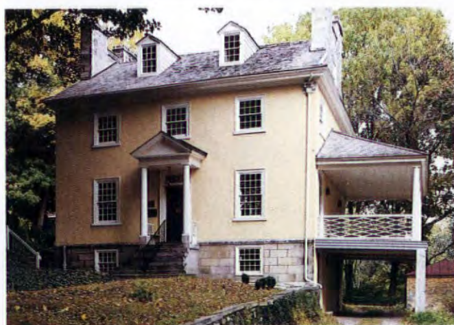
The Federal-style, stone and stucco house in 1990, after being repainted with acrylic latex paint.
