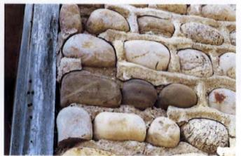
Mortar-joint failure in a cobblestone wall, possibly due to a bardness mismatch between original and repointing mortars.
