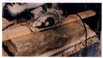
To level a stone face, run a circular saw along a  $2 \times 4$  with the blade set to the deepest depression in the stone.
