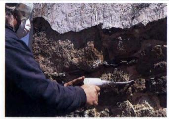
Careful use of a chipping gun removes old mortar, but some band chiseling is still necessary and does the job best.
