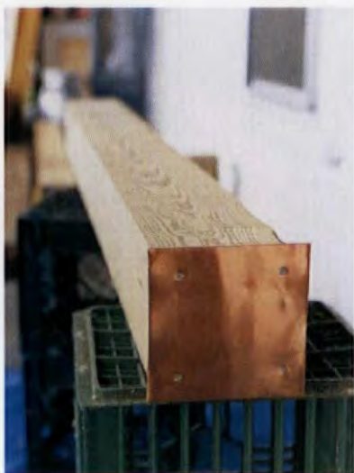
Flashing of 16-oz. copper at post bottoms protects wood from moisture.
