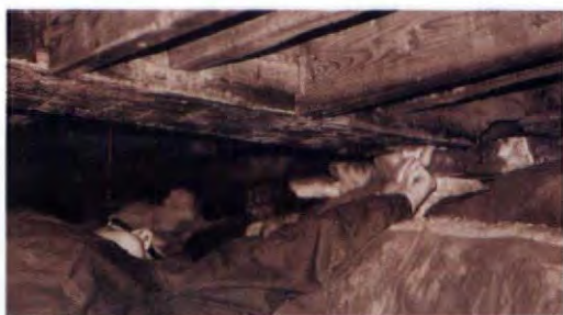
The sill in this damp crawl space has decayed where it joins a girder and is spongy enough to be punctured by a finger.
