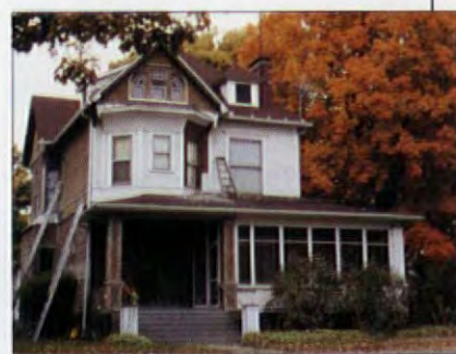
A house in Valparaiso in three stages of preparation: strip, sand, and prime.
