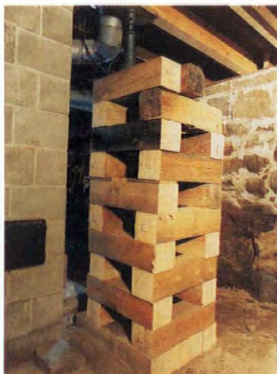
Because we were jacking three floors, we used 20-ton screw jacks and heavy timber cribbing to minimize risk.
