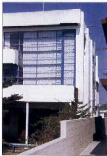
Schindler's Lovell Beach House is supported by concrete frames and stilts. (Newport Beach, Calif., 1926)
