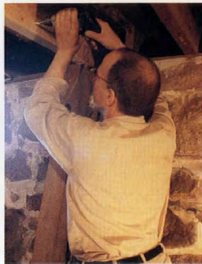
We drilled through the old joist, using the predrilled holes as a template to ensure that the rod holes would line up without the need of a long bit.
