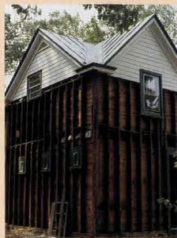
Only the joist ends and fire stops mark the second floor of this balloon-framed stable in Richmond, Virginia.
