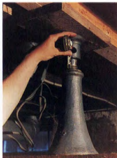
How much to jack? Measure initial thread exposed plus the amount you want to raise the floor plus 1/4-in.
