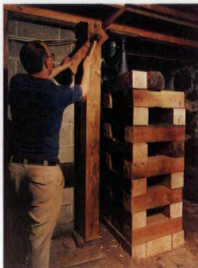
The permanent post should go in easy, with only moderate taps.
