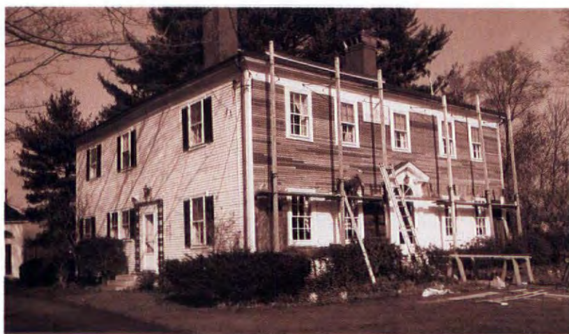
Reclapboarding an Adam house exposed a damaged sill and a whole new project.
