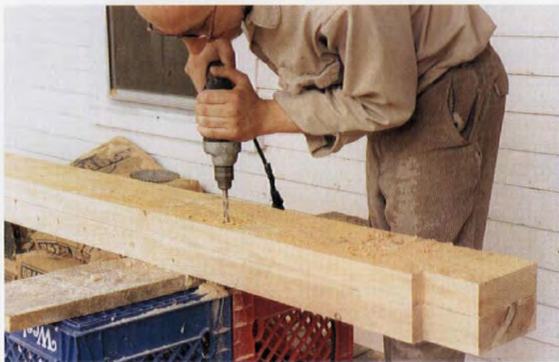
New reinforcement timbers were stacked and predrilled for the threaded rods that would hold them to the inadequate original joist.
