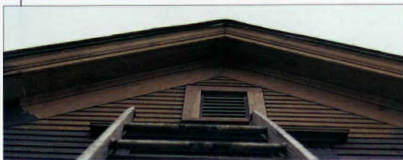
The dangerous, uppermost gable of the "Stormy," partially stripped and sanded to reveal like-new wood.
