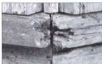
This rotted - and irreplaceable - woodwork...
