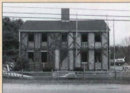
A c. 1815 timber-frame house, sans siding. Note the extensive wind bracing needed for this seacoast site. Photo by John Leeke.
