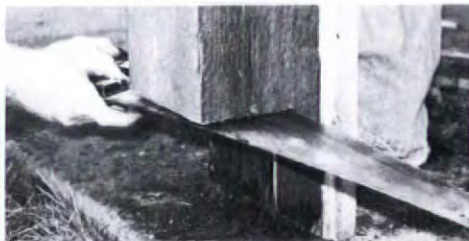
10" rotted bottoms of these load-bearing columns...
