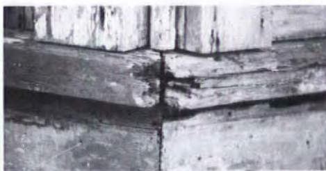
This rotted – and irreplaceable – woodwork...
