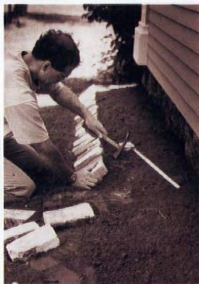
Laying the drip course: contractor Mike Tero digs a furrow and then tamps bricks into place
