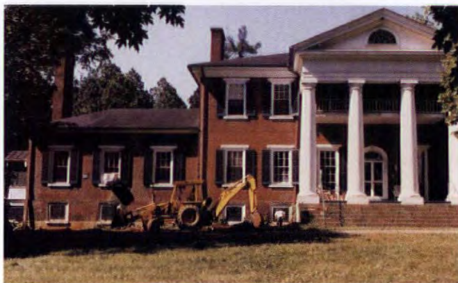
The backhoe begins excavation near the foundation of this Jeffersonian Greek Revival.
