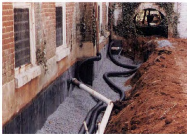
The Bituthene asphalt/polyethylene membrane in place, with a temporary downspout line visible.
