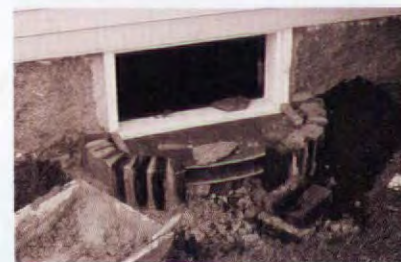
Top photo shows the anachronistic (and less enduring) galvanized window well. A better idea: New clay layer is tamped down, sloped away from foundation. Next, plywood form edges guide curve of brick course. Then the bricks are laid up in mortar to form an arched soldier course.
