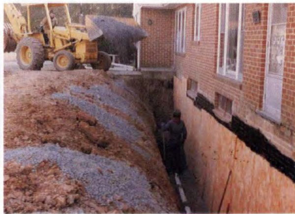
Tuff-N-Dri in place with protection board. Rigid perforated drain pipe is being bedded in gravel.
