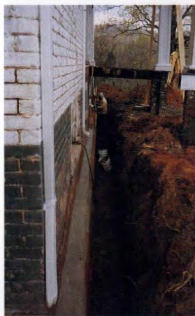
Top, the foundation wall is cleaned with high-pressure water before parging. Middle, note the unevenness of the wall below grade. Above, the brick foundation is parged (plaster-coated).
