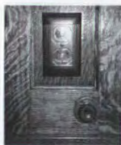
Call-bell plugs (above) were wired to push buttons (below) that clipped to table legs.
