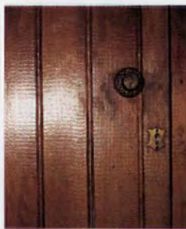
Note the uniform, wave-like ridges (knife marks) on these cylinder-planed boards.
