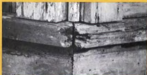
This rotted – and irreplaceable – woodwork...
