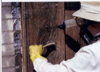
An alcohol rinse removes the last residue of chemical remover while masking protects the adjacent surface.
