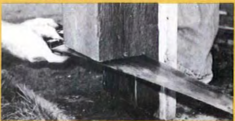
10" rotted bottoms of these load-bearing columns...
