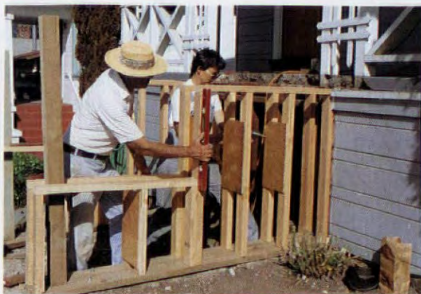
Each wall was two 2x4 frames tied together with plywood. Sills were treated lumber anchored to the old masonry footings.
