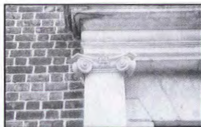
Capital replacement using Jahn Dry Casting Mortar (M150), Pohick Church, Lorton, VA
