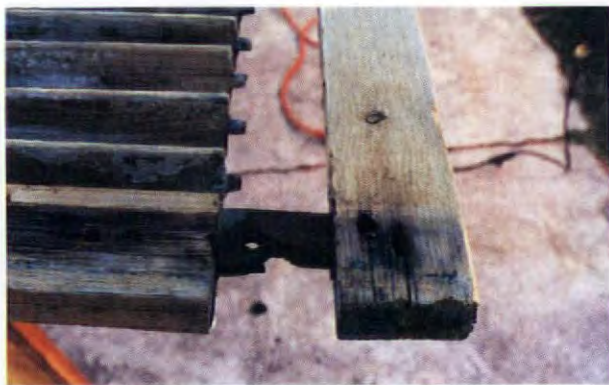
As the first step in restoring movement to stuck vanes, we tapped one side of the frame apart and gently worked the vanes out of their sockets.
