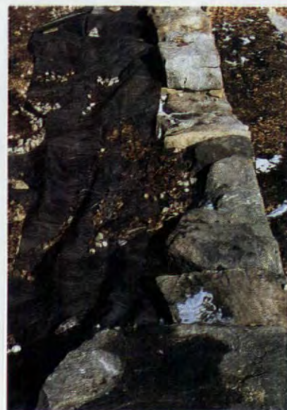
Landscaper's black filter paper is placed over the backing of a wall ready for topsoil.
