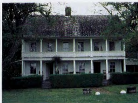
Planks in the 1856 Charles Applegate house in Yoncala, Oregon, rise as one piece for two storeys.
