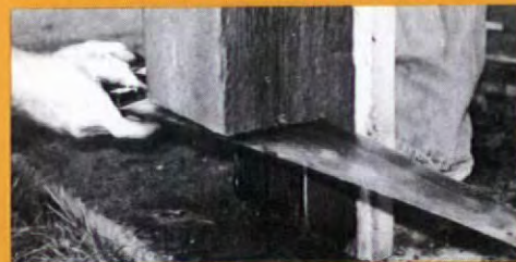
10" rotted bottoms of these load-bearing columns...
