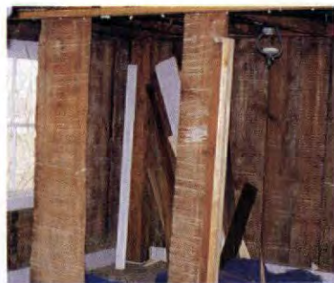
Random-width planks — some the diameter of a tree — also partitioned interiors.
