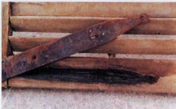
(above) The horizontal edge of the hinge retarded drainage, and condensation behind it contributed to wood rot. When it was necessary to add to previously hardened filler (below), we roughed up the surface thoroughly with a knife or nail and coarse sandpaper.
