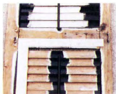
We used a hand-held drill bit to ream the old paint out of the vane holes, and cotton swabs to prime and to paint them. This provides a smooth bearing surface and protection from trapped water.
