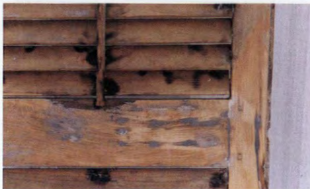
A prime coat of thinned resin consolidated the damaged wood and provided a strong surface for the filler to adhere to.
