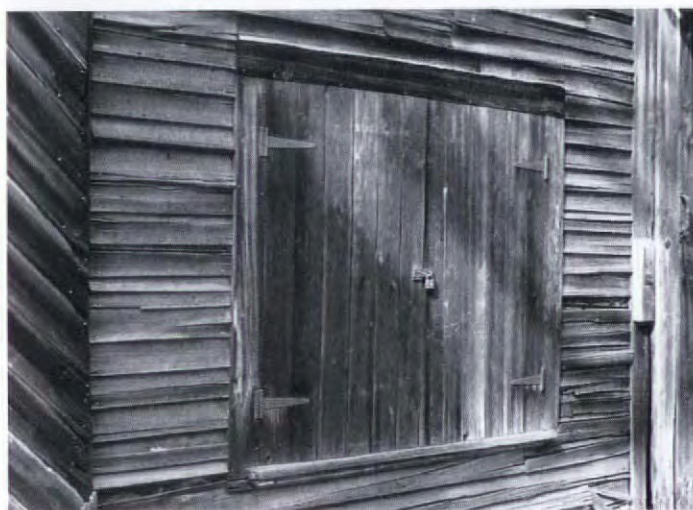
Shutters were often homemade from several boards joined on the back by horizontal battens.
