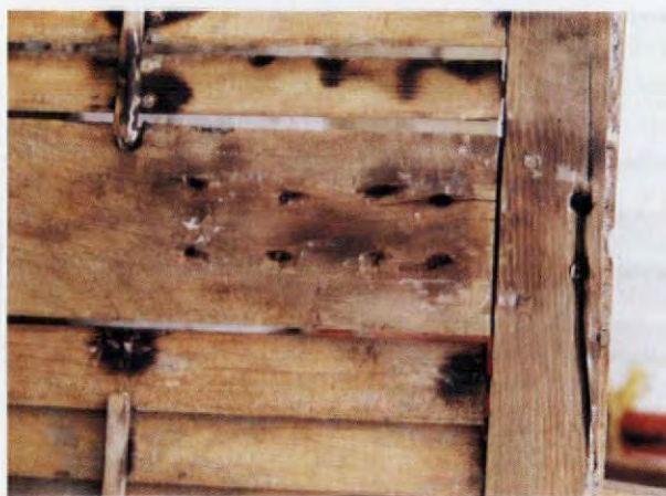
Stripped shutters revealed their problem spots. On this one, standard repair attempts of plugging screw holes with wood had failed and left holes, some as large as 1/2" in diameter.
