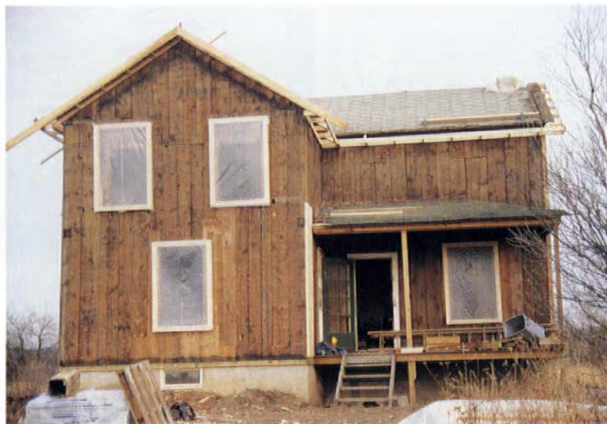
Siding off, the vertical planks supporting this house without corner posts become clear. Note the joist pockets near the windows.
