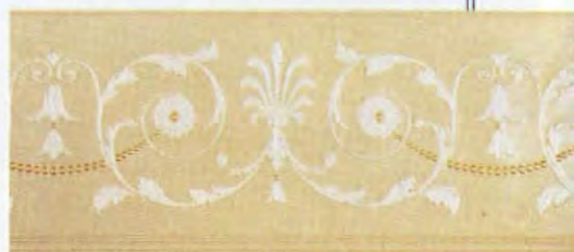
Simple but effective: White paint on raised areas simulates plaster decoration; the beaded swags were "gilded" with Dutch metal.
