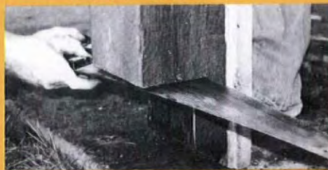
10" rotted bottoms of these load-bearing columns...
