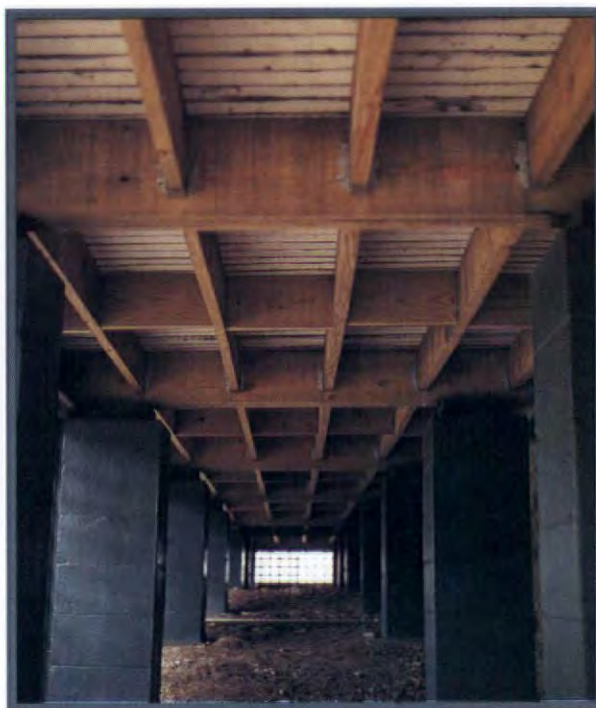
An under-deck view reveals deck boards protected with white primer backpainting and caulk at joints. Pressure-treated framing lumber stands up to high moisture levels near the ground.
