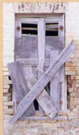
A common — but inappropriate — method of closing in that is as ineffective as it is unsightly.
