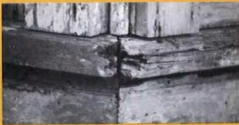
This rotted – and irreplaceable – woodwork...
