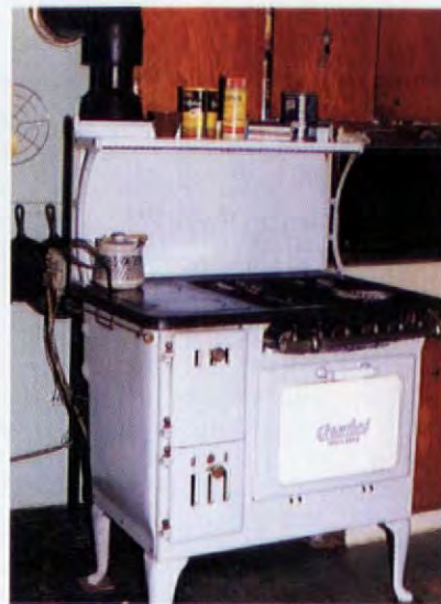
The firebox of a combination wood/gas range requires a safe clearance from combustible materials.
