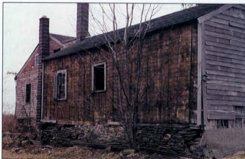
The vertical plank construction seen under the clapboards of this Ithaca, New York, house is a technique found across North America.
