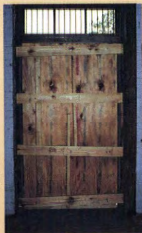
Multiple stud lumber strongbacks on a door interior. Transom vents were already present.
