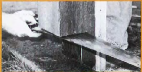
10" rotted bottoms of these load-bearing columns...
