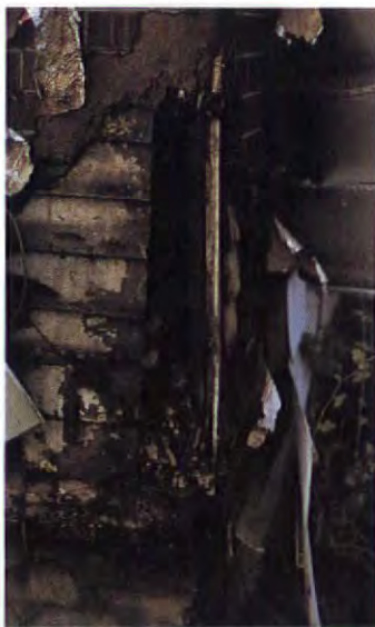
Three layers of material are peeled back to expose a hole that used to be the corner post.
