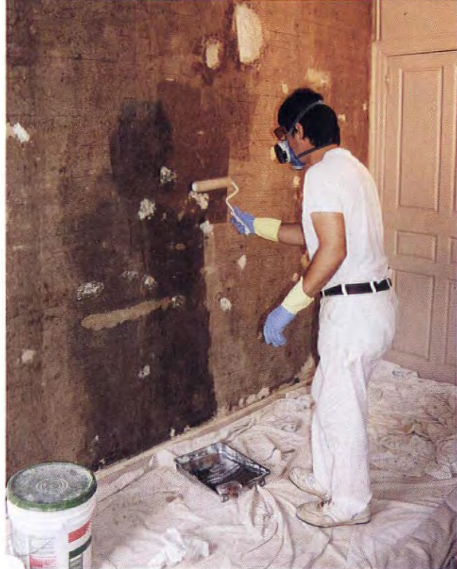
Peter applied our consolidant mix in three coats, using a bristle brush for edges and a roller for fields.
