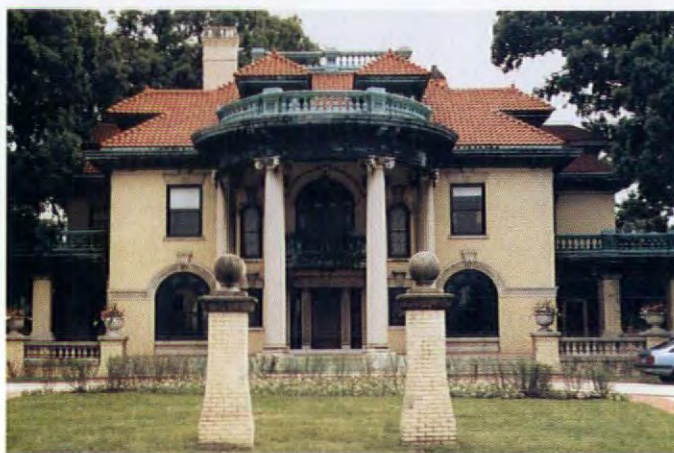
The stained copper balustrades and cornices of this Mediterranean-style mansion may respond to chemical cleaning or "agri-blasting."
