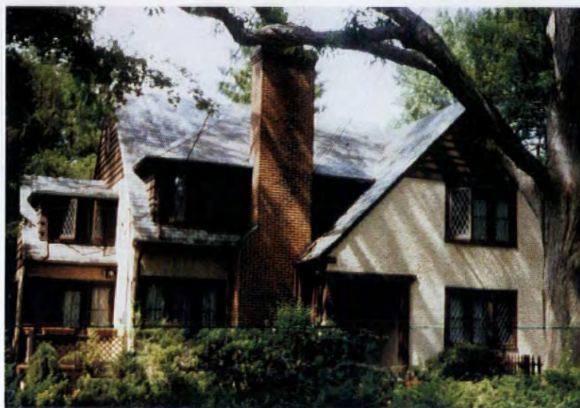
Stucco, leaded casement windows, front-facing chimney, and steep roof lines key the Lemkes' 1920s house as English-style in the American suburbs.
