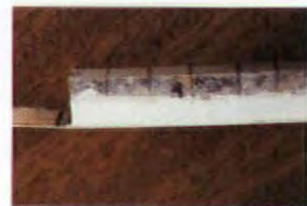
This bead moulding from a mid-19th-century baseboard shows the precise hand-cutting needed to kerf the piece close to the rounded profile.
