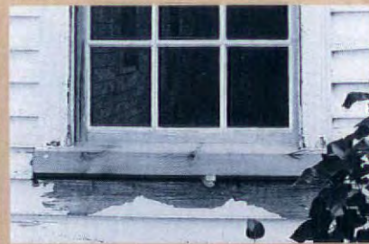
▲ The new sill replaces the original which was severely decayed due to water entry.
