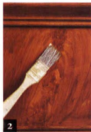
2 Immediately blob an extra amount of the glaze down the middle of the U.
