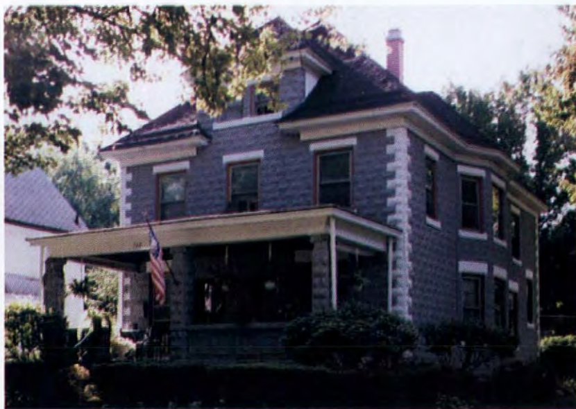
Concrete block construction was pushed as an ideal small business by equipment makers, spawning thousands of houses like this c.1910 Foursquare.
