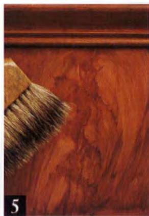
5 As the glaze begins to set up, soften your work with a blender by brushing diagonally across the surface.
