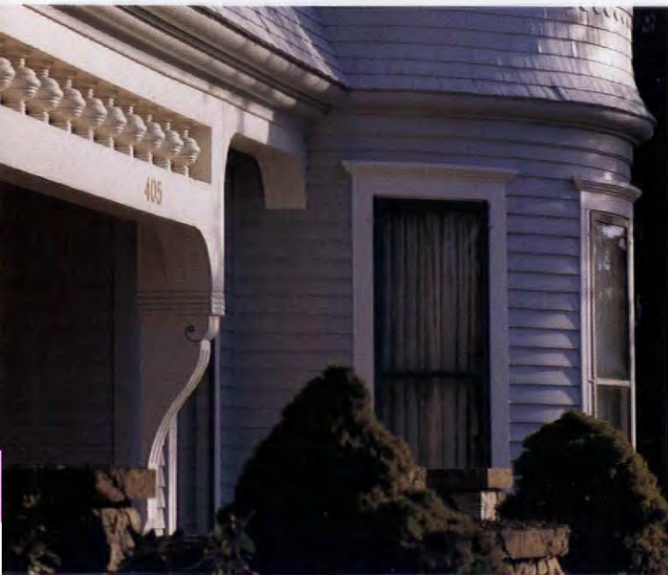
Beveled clapboards are common siding on circular towers and walls, but in order to lay horizontal they must be cut in an arc.
