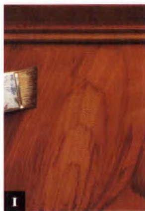
1 Apply the glaze in an upside-down U-pattern.
