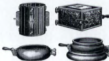
Fluted columns, piers, rings, and bases were just four concrete molds from the Sears "Porch Outfit."
