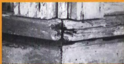
This rotted – and irreplaceable – woodwork...
