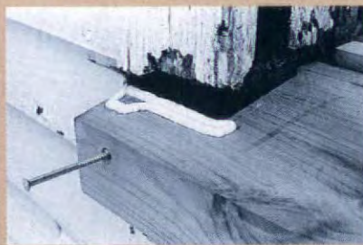
▲ Sealant is applied on the top surface of this new sill where the end of the facing board will sit. After installation, the countersunk screw hole is filled with sealant.
