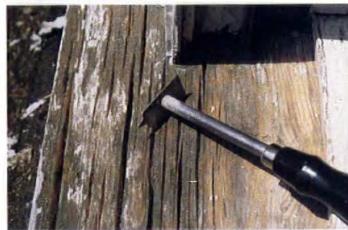
Before treating, deep weather checks can be cleaned with a scraper made for the purpose.
