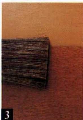
Slap diagonal pores into the wet glaze with the flogger. (This also can be done last.)
