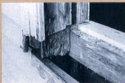
▲ Removing the sill exposed decay in this dado joint at the lower end of the frame stile.
