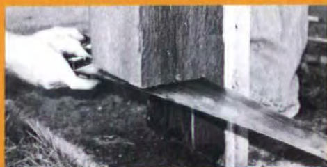
10" rotted bottoms of these load-bearing columns...
