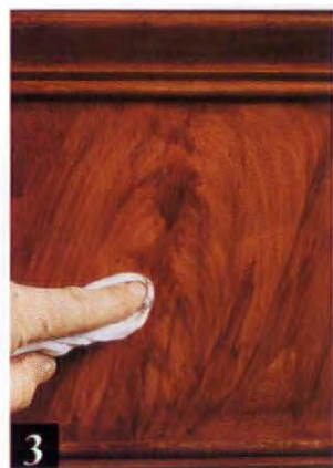
3 With a rag, wipe out highlights from the center, avoiding symmetry.
