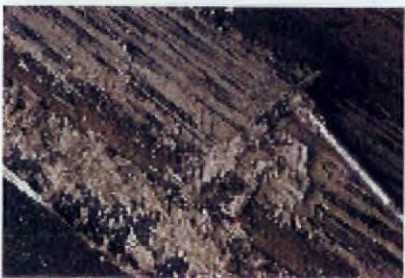
(top) Priming checks with epoxy consolidant. (middle) Working epoxy filler into checks. (bottom) Scraping away excess filler.
