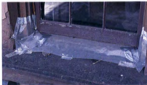
Poly sheeting keeps the sill dry and flips up for work.
