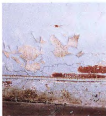
Peeling paint and plaster, along with musty smells, are classic symptoms of rising damp.
