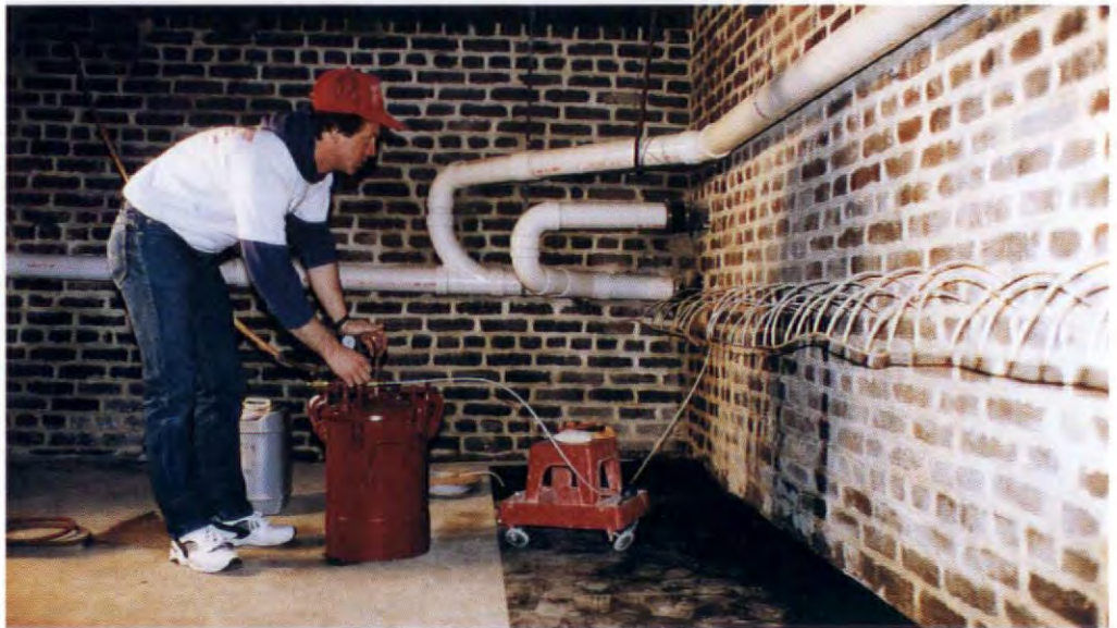
Top: Chemical damp-proof course processes and materials vary, but all inject resins through many small holes. Right: Cutting for a mechanical damp-proof course is tricky, expensive, and limited to certain wall types.
