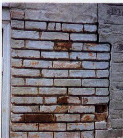
Resurfacing involves clearing mortar joints as if repointing, and then filling voids in brick.
