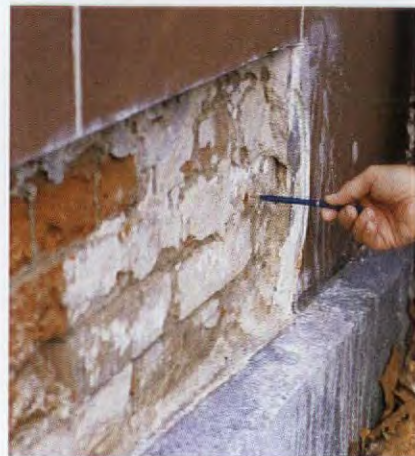
Removing plaster revealed a rising damp condition; keeping it off promoted evaporation.
