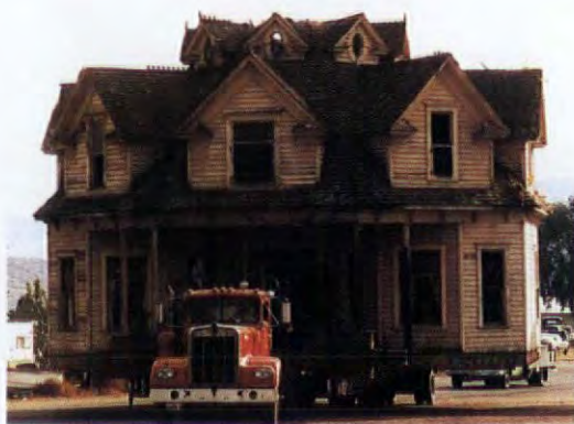
Relocating Cecile Allen's octagon house required removing its steeple-like roof tip in order to clear power lines.
