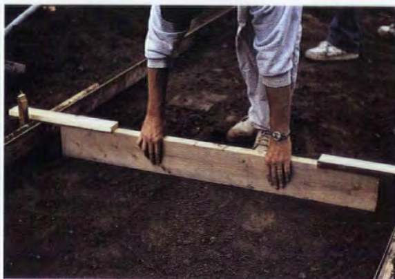
As it is pulled along the forms, the 6" screed board levels the earth, which is now ready for a layer of stone dust.
