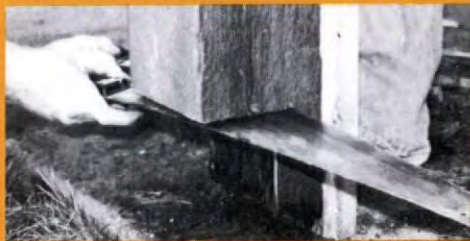
10" rotted bottoms of these load-bearing columns...
