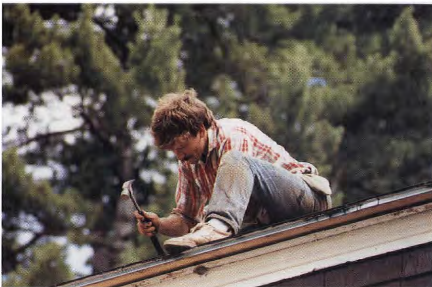
Loose shingles, ice dams, and holes punched by branches kept us busy on the roof more than once over the years. Here Curt is working on the first reshingling project.
