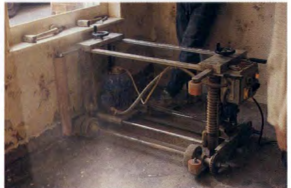
Top: Chemical damp-proof course processes and materials vary, but all inject resins through many small holes. Right: Cutting for a mechanical damp-proof course is tricky, expensive, and limited to certain wall types.
