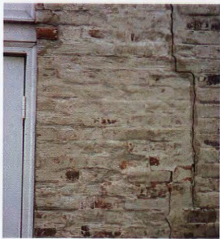
Chipped brick, sloppy repairs, and gooey overcoats can mean repointing is not enough to resurrect the wall.
