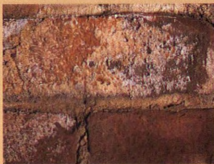
Efflorescence — a sign of moisture.
