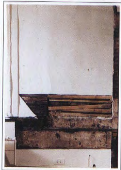
FIG. 3 EXCAVATING THE PLASTER
