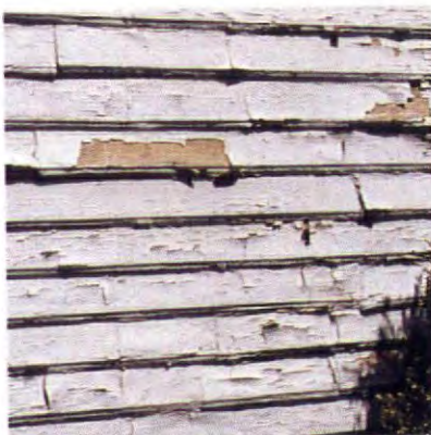
Peeling down to bare wood
