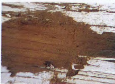
Sand weathered areas until “bright” wood shows.
