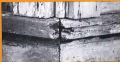
This rotted – and irreplaceable – woodwork...
