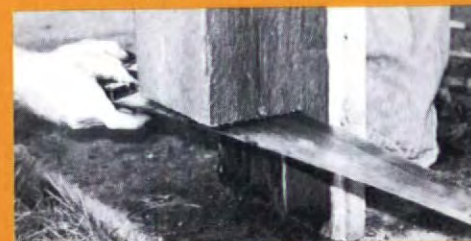
10" rotted bottoms of these load-bearing columns...
