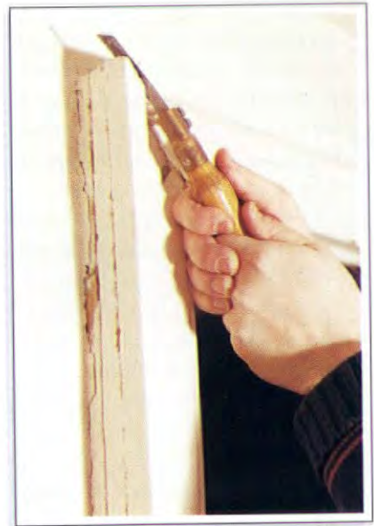
FIG. 1 SLICING NAILS
