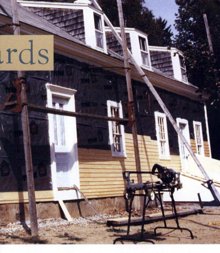
updating the mechanical systems. While removing all the exterior shingles and sheathing in order to check framing and install wiring, we discovered evidence that helped Chris and Becky decide on the type of new siding.
