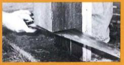
10" rotted bottoms of these load-bearing columns ...
