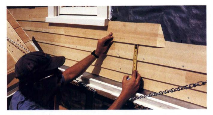
Clapboards usually have to be fitted into the sill siding groove, often with some fudging of later course exposures.
