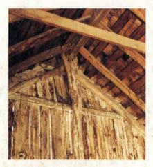
A jacal (top) survives in Los Saenz, Texas, under a new wood shingle roof. A natural fork in the end post supports the ridge pole of a typical 12' by 18' jacal (above).
