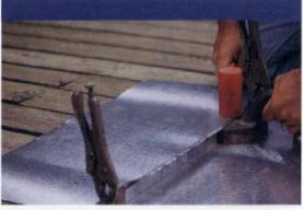
The author demonstrates the first fold of the seam. Work as far along as possible between locking pliers.
