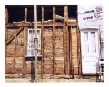
Removing later siding and original sheathing boards exposed the structural frame for inspection and wiring. Note the split-board lath and plaster.
