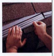
Install the Shingle Shield under a course of shingles on each side of the ridge.
