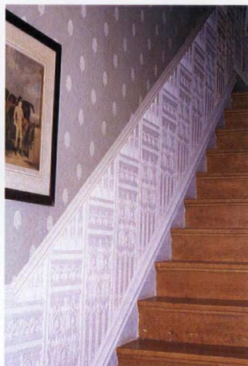
The completed installation of an Edwardian Lincrusta dado. Note how the extra triangular piece is fitted above each half panel and then finished with a length of chair rail moulding.
