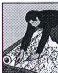
1. Cut fiberglass mat 2" longer than height.
