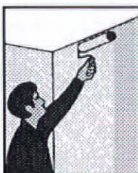
2. Apply saturant to area to be covered.
