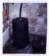
TOP: Cracks in concrete should be sealed with urethane caulk. MIDDLE: Fill penetrations in first-storey floors with radon-blocking foam. BOTTOM: A sump pump cover ventilates ground-source air from the pump to the outside.
