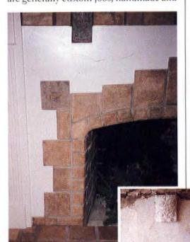
Often restorations requires replacing tiles with replicas. In this case, however, the painted ornamental tile was cleaned and the damaged field tiles on the fireplace surround were repaired.
