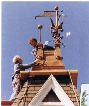
new roof. A "hollow" rectangle of staging lumber, held together with carriage bolts, and flipped over the top of the tower like a ring toss, did the job. We'd simply unbolt the corners and lower the pieces on safety lines to remove it after the weathervane was in place.
