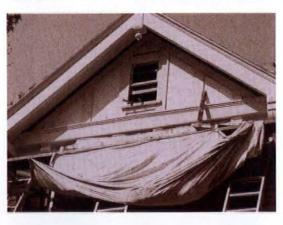
Top: To prevent costly mistakes, cut out windows after the canvas has been stretched over most of the gable. Middle: Completely tacked into place, the canvas is heavily coated with primer. Bottom: Once the canvas is dry, install the rakeboards to tighten it and then follow with the wood trim.
