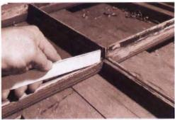
of the sash. I like to make this a press fit so the part holds itself in place during gluing. To get this fit, I cut it long and trim the length with a sharp chisel or sandpaper. I use epoxy adhesive formulated for use with wood, or a mixture of epoxy consolidant and epoxy paste filler. If fasteners are needed, use wire brads.
