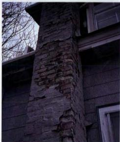
TOP: Creosote on the exterior of the chimney means big problems: condensation, interior creosote buildup, and deteriorated masonry. ABOVE: Sometimes soft brick was used to build chimneys. This masonry does not stand up well to flue gases or weathering.
