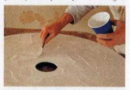
Make sure to get a good, thick coat of adhesive on the back of the run surround.
