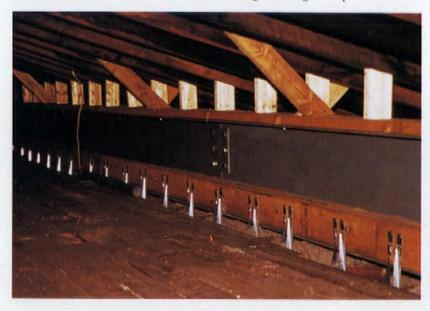
were bolted together, they formed two 35' beams that ran the length of the attic.
