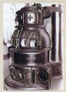
Special piping behind the Baltimore Heater reburned exhaust and ducted heat to upstairs bedrooms.
