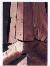
FAR LEFT: Cleats provide anchors without penetration and give the metal freedom to move. MIDDLE: If you're replacing flashing on an existing roof, you'll need to remove adjacent roofing. LEFT: The bottom edge should be doubled under and formed into the gutter system.
