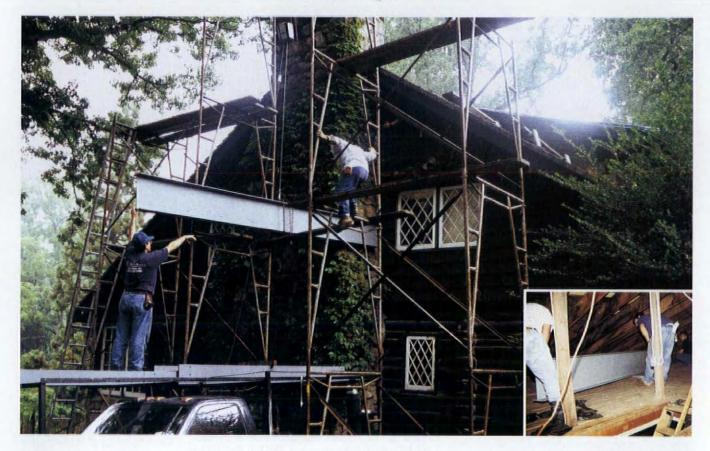
ABOVE: An attic vent window (above worker in photo) provides a way into the main building for the dormer steel. INSET: More pipes position the steel once inside. BELOW: Now in place, one two-piece dormer beam is connected to the the existing framing by cripples and fasteners.
