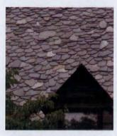
Specifying staggered butts, staggered exposure, and clipped corners can take the textural roof to an extreme level, producing a crazy guilt of slates.
