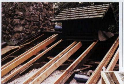
**ABOVE: The kitchen rafters** had spread worst at the middle of the roof - so much so that they affected how the roof tiles drained. Sistering with 3 x 8 lumber reinforced each rafter with identical material, but was not intended to correct the sag. INSET: The sisters stopped short of the original rafter tails, which were restored with epoxy fillers.
