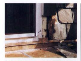
Flashing must be integrated into the roofing and compatible with adjacent materials.
