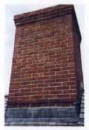
Skillful repointing looks just like the existing masonry. New mortar and replacement brick must match the originals.
