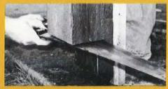
10" rotted bottoms of these load-bearing columns.
