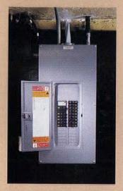
This modern service panel, with all breakers in a single enclosure and labels on the inside door, is easy to understand in an emergency.
