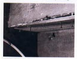
Cabinet-grade power drive screws are well adapted for riser repairs. However, make sure the load is against the head—not the shankof the screws. Some screws, especially those made for drywall, may fail under shear loads.
