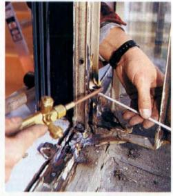
Make sure the metal frame is strong enough to anchor the hinge. Then weld it in place, taking care to position it properly.
