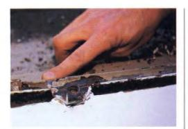
Weep holes should be opened up so that water can drain to the exterior.
