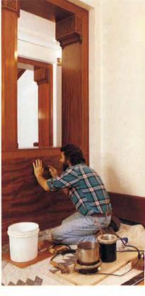
Steve Hirschfeld, Traditional Line's senior wood restorer, perfected the repair of the veneer "bubbles". First, he heats the diluted hide glue mix in an electric "glue pot" (above). Bubbles are held open with an artist's palette knife while the glue mix is injected (Fig. 1). An electric iron helps re-adhere the existing glue (Fig. 2). Rolling presses the bubble flat and holds it down until the glue sets (Fig. 3).
