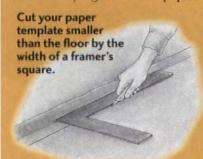
at the edge of the floor, where it can be difficult to maneuver and where the blade can damage fixtures, place a framer's square on top of the paper and against the edges of the floor. Then cut the template along the inside edge of the square. The result will be a mockup that is scribed 2" smaller than the floor area, but which was much easier to create than the entire floor would have been. When transferring the model to the linoleum, simply use the framer's square again, adding its width.
