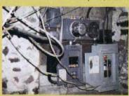
The electric service panel at the Hitchcocks' new house was charred and fastened to a rotting board.
