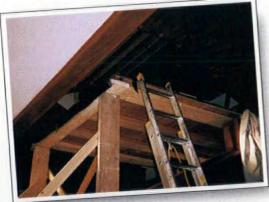
Steve had to assemble a scaffold to re-install the heavy stair panels. We placed packing blankets in strategic spots, then a gang of able bodies—with freshly washed hands—lifted the panels back up into their original positions for fastening.
