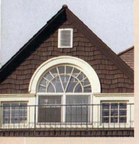
Shingles that produce shape effects (such as diamonds and waves) with decorative butts were on the wane by the time this Shingle-style house was built. The new popularity of stains made texture and course patterns more appealing.
