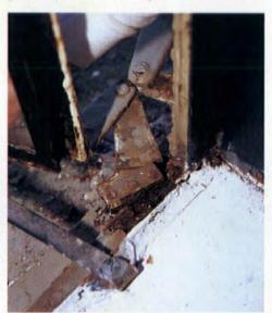
As the vents are being aligned, the contractor should check the hinges. They may have rusted and come loose from frames or vents.
