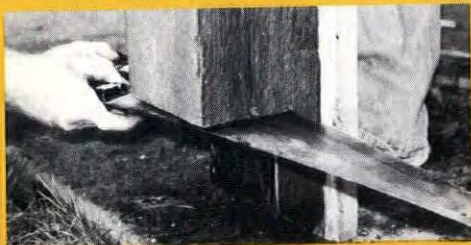
10" rotted bottoms of these load-bearing columns...
