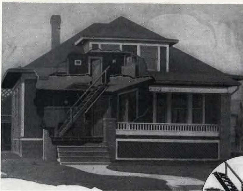
Many a disappearing-stair company built its business on bungalows by saving space downstairs or opening the attic for living. Inset: Disappearing stairs that do not collapse in some way feature continuous stringers that slide down to the floor and tip back into the attic.
