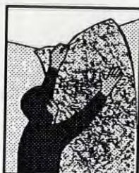
3. Apply fiberglass mat to wet surface.
