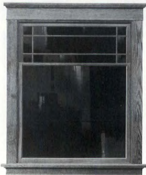
Cottage front sash (left) made use of a high-waisted meeting rail. The heavily horizontal accent of this nine-light pattern was a classic with many foursquares and bungalows.
