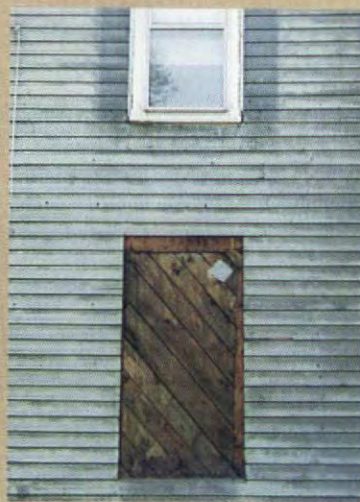
The diagonal sheathing on the house runs uninterrupted through the window opening, and an original staircase is on the inside.
