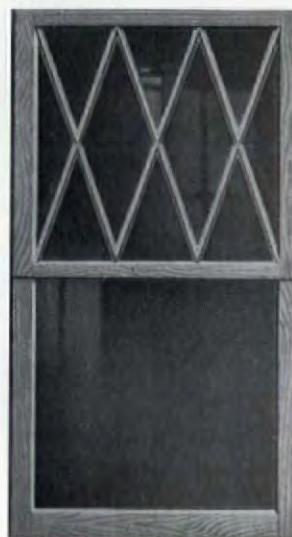
Cottage front sash (left) made use of a high-waisted meeting rail. The heavily horizontal accent of this nine-light pattern was a classic with many foursquares and bungalows.
