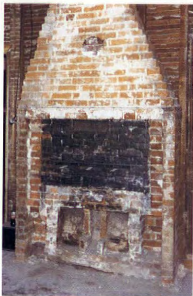
The only hint of this fireplace behind a plaster wall was the stove thimble.
