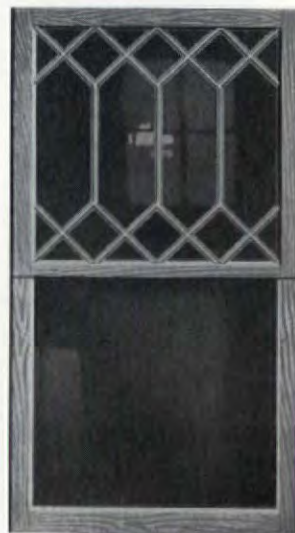
Cottage front sash (left) made use of a high-waisted meeting rail. The heavily horizontal accent of this nine-light pattern was a classic with many foursquares and bungalows.
