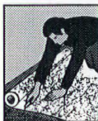
1. Cut fiberglass mat 2" longer than height.
