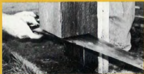
10" rotted bottoms of these load-bearing columns...
