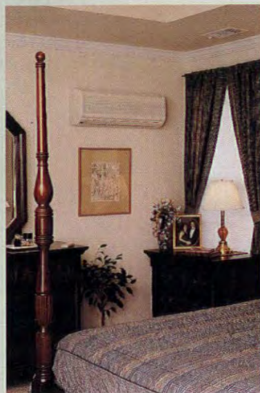
Although undeniably modern in an old house, the ductless system has very little physical impact on the historic structure.
