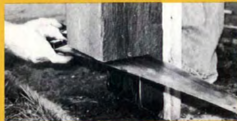
10" rotted bottoms of these load-bearing columns...
