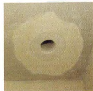
Top: The best outlet locations are in the ceiling at each corner along the exterior wall, but this may not always be an option. Middle: The duct blows cold air into the corner of the room where people rarely stand. Above: You can feather the plaster surface with joint compound to hide the flange.
