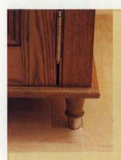
Reproductions of original cabinet legs created a toe space and kept the 19th century look (above). However, actual support came from plywood bases that could be leveled and trimmed out before installing cabinets (below). Carefully taped particle board protects the floors.
