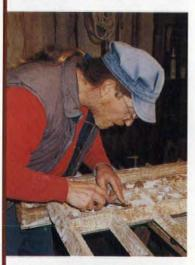
Co-author Thomas Glynn chips loose paint from a quatrefoil in the SPNEA workshop in South Berwick, Maine, where fence sections were repaired and rebuilt piece by piece.
