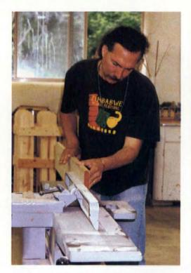
Carpenter Mark Sabella fabricated new cabinet doors, made 3" taller than the originals so as to cover the extension joint (right). Proportion and detail follow existing cabinetwork in the house (below right).
