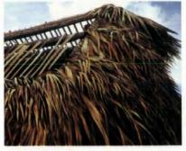
Originally tied to the frame with fiber or bark cordage, fronds are now usually nailed in place.
