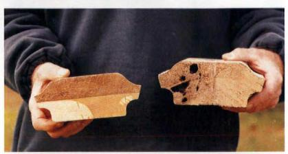
using epoxy fillers (see "Better Than Wood," p. 56). Since similar rail stock was all but impossible to find, we created new stock by sandwiching two pieces of roughly dimensioned lumber. The white pine boards were doweled and glued with an adhesive epoxy, clamped together, planed to the rough dimensions needed, then sanded smooth.
