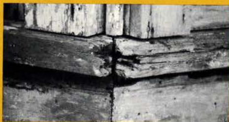
This rotted – and irreplaceable – woodwork...
