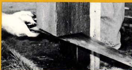
10" rotted bottoms of these load-bearing columns...
