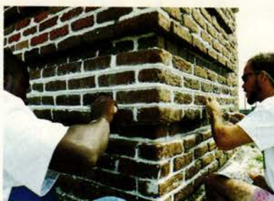
Participants in a masonry workshop perfect the finer points of V-joints.
