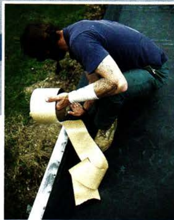
Above: With EPDM seams of all kinds, the first step for a good seal is cleaning the membrane of powder. (During the rolling process, manufacturers apply either mineral talc or mica to the rubber so sheets won't stick to each other.) Right: Metal flashing is one option for terminating the membrane at roof edges. Butyl tape, which is extremely sticky, completes the job.
