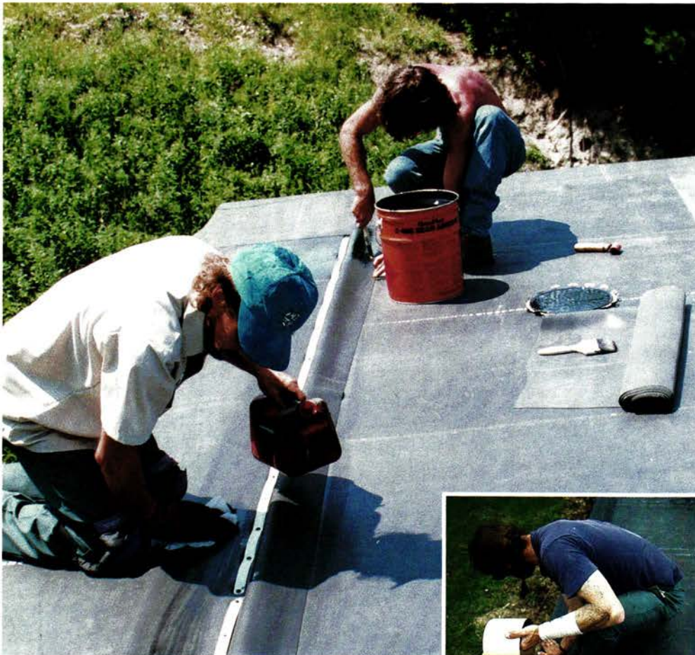
Above: With EPDM seams of all kinds, the first step for a good seal is cleaning the membrane of powder. (During the rolling process, manufacturers apply either mineral talc or mica to the rubber so sheets won't stick to each other.) Right: Metal flashing is one option for terminating the membrane at roof edges. Butyl tape, which is extremely sticky, completes the job.
