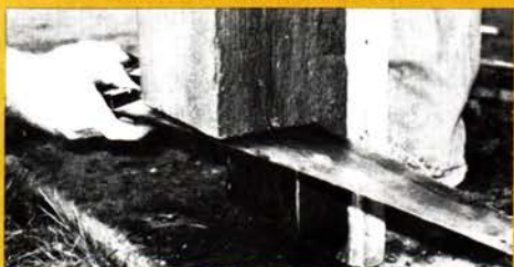
10" rotted bottoms of these load-bearing columns...
