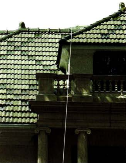
French tile was invented in the 1890s, making it a suitable choice for a Neoclassical dwelling. The diamond pattern above was created by combining Ludowici tiles in two different shades of matte and glazed green.
