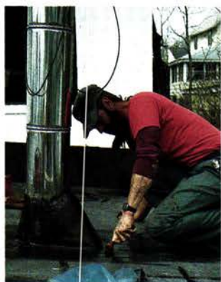
Vents and other penetrations are made watertight by fitting patches of uncured EPDM (top), then rolling and coating with sealer (above).
