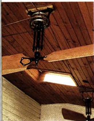
Rotary fans move the air at a leisurely 60 to 100 rpm.
