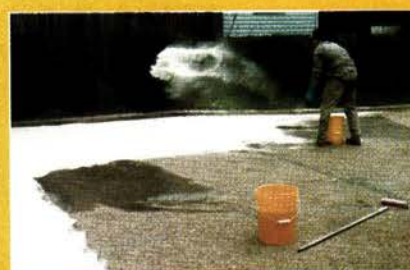
Grit being applied to restored driveway
