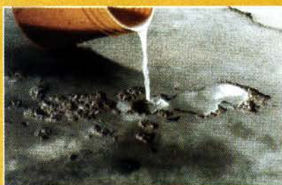
ABOCRETE repairs and resurfaces spalled concrete.
