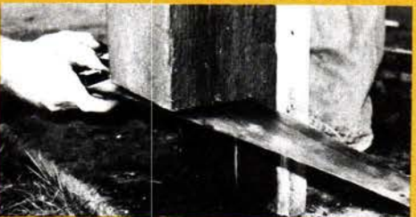
10" rotted bottoms of these load-bearing columns...
