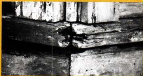
This rotted – and irreplaceable – woodwork...
