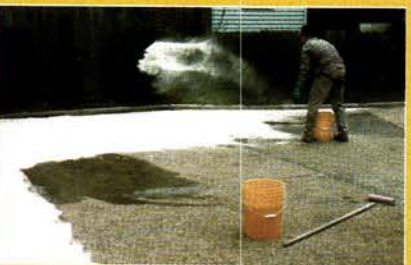
Grit being applied to restored driveway
