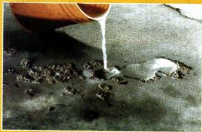
ABOCRETE repairs and resurfaces spalled concrete.
