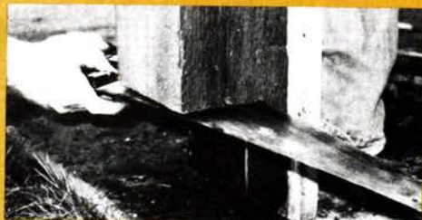
10" rotted bottoms of these load-bearing columns...
