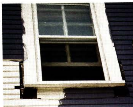
The cavities surrounding this casing are evidence of decorative window frames—exactly in step with the Italianate style.
