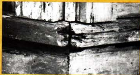
This rotted – and irreplaceable – woodwork...
