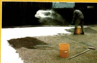
Grit being applied to restored driveway
