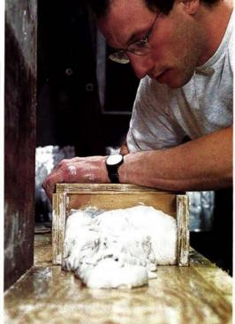
Left: As Frank lays the first batch of plaster, it pours out of the bucket at roughly the consistency of cake frosting. Above: Part of the skill of running the mould is keeping the two vertical slippers in constant contact with the bench and tight against the lattice (right in photo) while it pushes through the slippery plaster.
