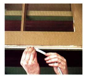
Rubber bulbs and seals are effective for sash window bottoms, but may require power tools to cut the kerf that holds the barbed flange.
