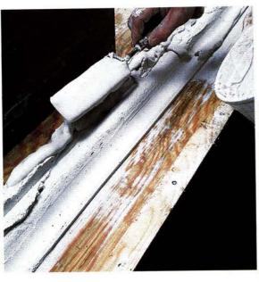
Top right: To fill the surface for the final runs, Dave points out minor blemishes and craters while Frank brushes them with soupy plaster. Another pass or two of the knife with a "baptizing" of water give the moulding its finished polish.
