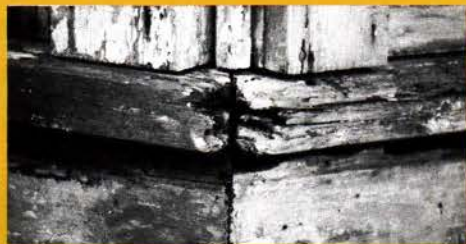
This rotted – and irreplaceable – woodwork...
