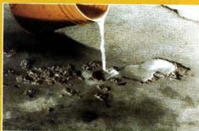
ABOCRETE repairs and resurfaces spalled concrete.
