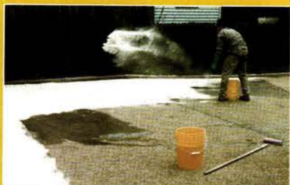
Grit being applied to restored driveway
