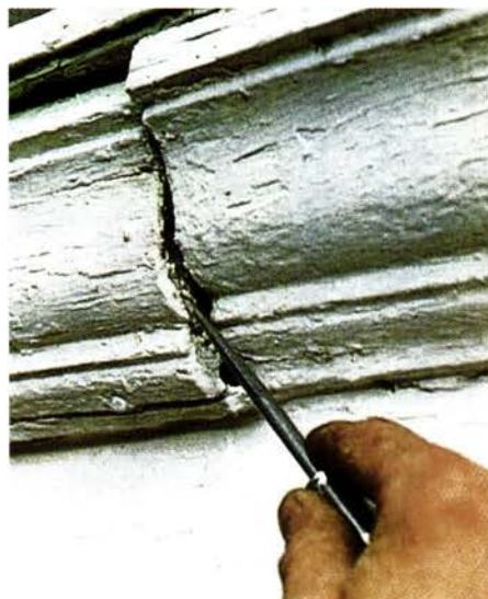
Exterior wood deterioration: a leak in the flashing caused nails to rust, which opened this joint in crown moulding. Rainwater now soaks into endgrain, causing decay.
