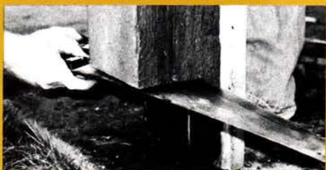
10" rotted bottoms of these load-bearing columns...
