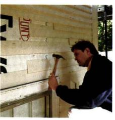
Clockwise from top left: Clapboards join in a mating bevel, nailed at each side. Hefty boards fastened with stainless steel nails make a weathertight finish for outside corners. In open areas, clapboards are carefully tacked in position to stagger joints. The siding starts with a beveled water table board; square sticks finish inside corners.
