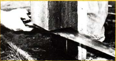
10" rotted bottoms of these load-bearing columns...
