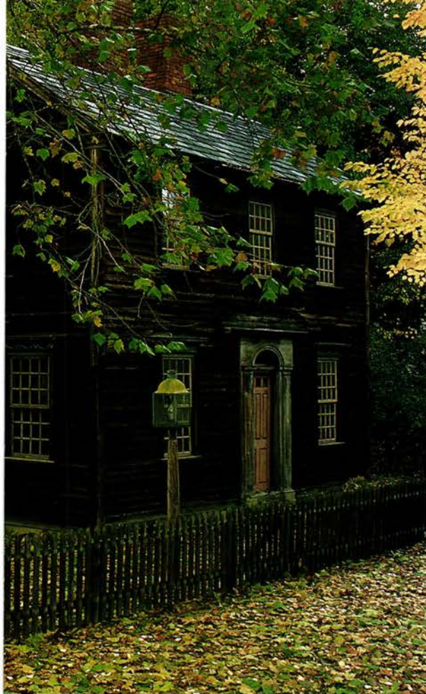
Whether wood or stone, the exteriors of early houses leave no questions about their structural system. The room-wide girth and regular bays of this 18th century house in Deerfield, Massachusetts belie the typical span of a timber frame.
