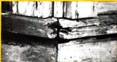
This rotted – and irreplaceable – woodwork...
