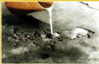
ABOCRETE repairs and resurfaces spalled concrete.
