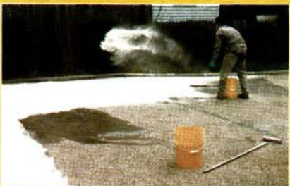
Grit being applied to restored driveway
