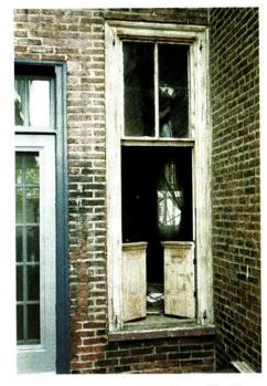
With the bottom sash raised, the combination door turns a window into an entranceway.
