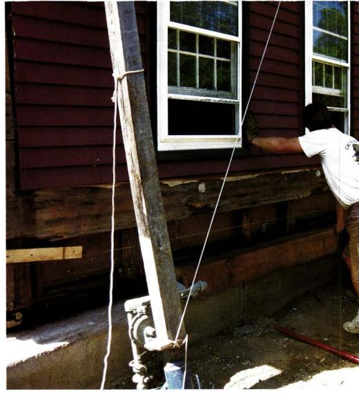
Sills may be the lowliest parts of a wood-frame house but, like the keel of a boat, they form the base that supports all other structural members. When old-house sills succumb to rot and insect damage, it takes technique and experience to replace them.
