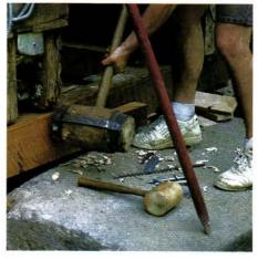
Left: George shoehorns in the new sill with a series of flatbars that ease joists and studs into place. Above: A swing of the beetle aligns the faces of the lap joint. Below: An electric lag gun, similar to an auto mechanic's lug wrench, drives in the lag screws.
