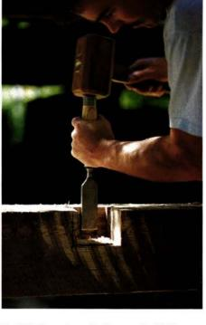
Far left: Measuring old sills reveals shrinkage from the original 8". Left: Hydraulic jacks on carefully angled pads suspend walls while George Yonnone and Curtis Von Ruden maneuver 22" of new white oak sill. Counterclockwise from above: A builders saw roughs out the old-style joist housings in the new sill; hole saws remove waste wood; final dressing with hammer and chisel.
